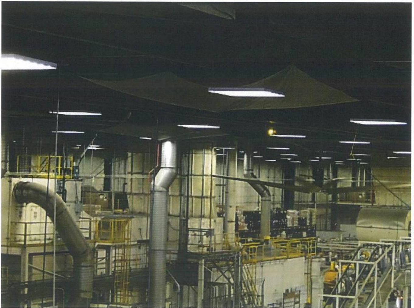
Photo #9721 View of tarps suspended from the roof structure at the Upper Roof Area to prevent roof leaks from damaging manufacturing equipment and products.
