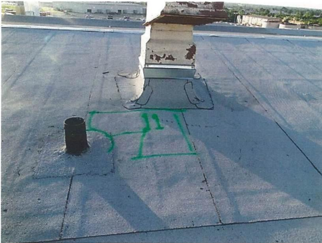
Photo #9702 View of entrapped moisture location #11 at between a plumbing vent and the rim of an exhaust fan curb at the Upper Roof near the east eave north of expansion joint #4.
