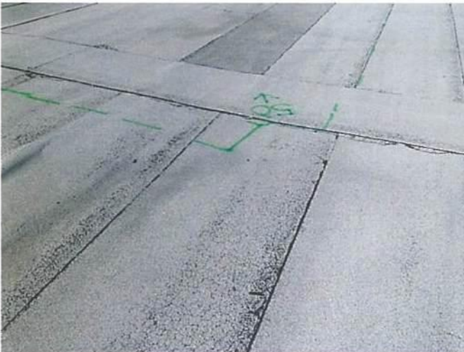
Photo #9774 View of entrapped moisture location #50 at the Upper Roof near the east valley north of expansion joint #11.
