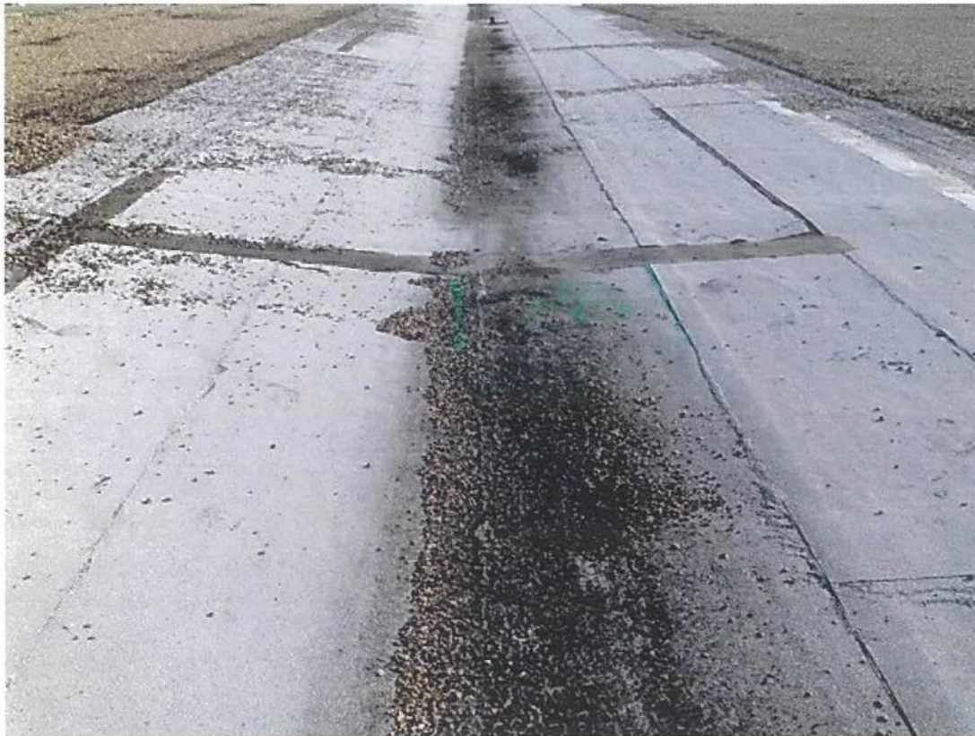
Photo #9766 View of area of entrapped moisture location #43 in west valley modified bitumen patch at the Upper Roof south of expansion joint #9.
