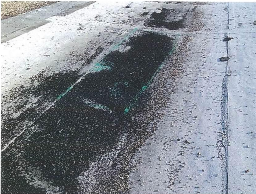
Photo #9752 View of entrapped moisture location #36 at the mineral surfaced modified bitumen roof patch at the east valley line of the Upper Roof north of expansion joint #8.
