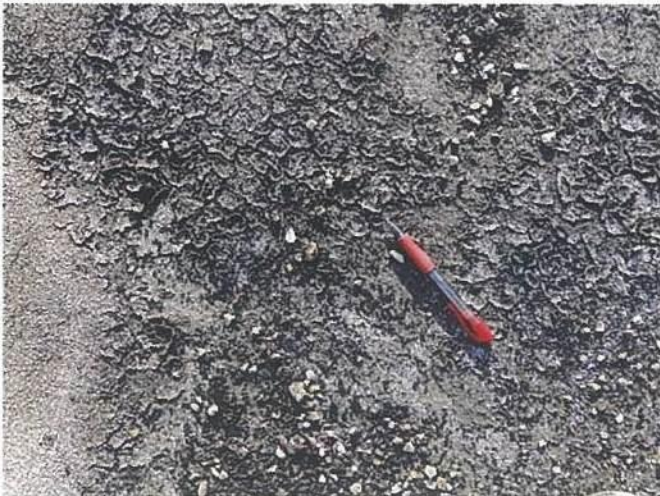
Photo #9761 View of delaminated mineral surfaced modified bitumen roof patch at the west valley north of expansion joint #8 at the Upper Roof due to long time exposure to ponding water.
