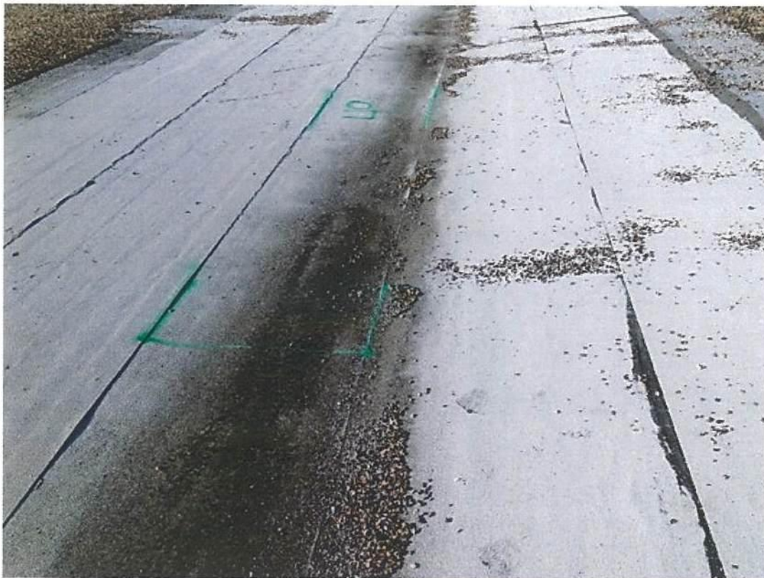
Photo #9765 View of area of entrapped moisture location #48 in west valley modified bitumen patch at the Upper Roof north of expansion joint #9.
