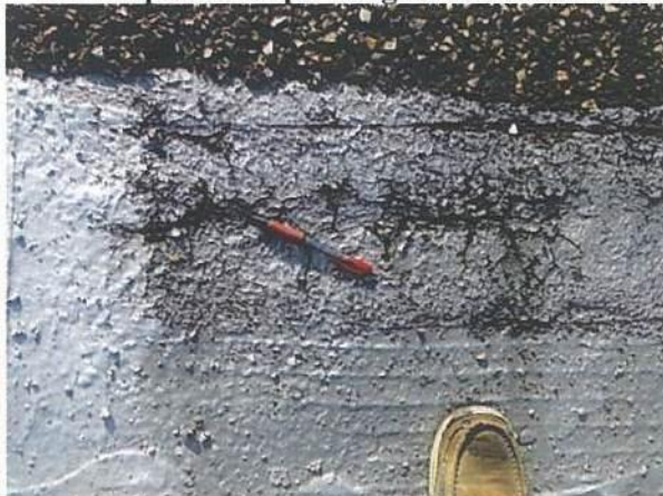
Photo #9767 Split Built-Up Roof near valley.
