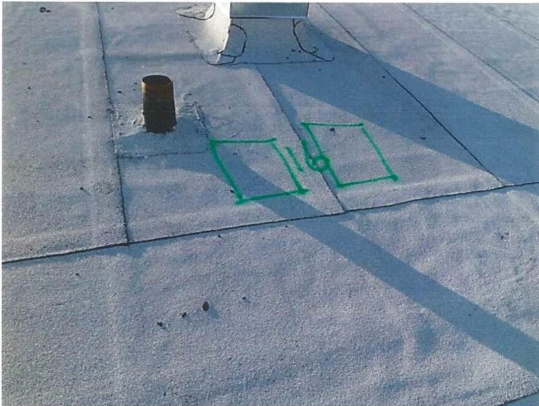
Photo #9708 View of entrapped moisture location #16 near base of an exhaust fan curb and a plumbing vent at the east side of the Upper Roof south of expansion joint #6.
