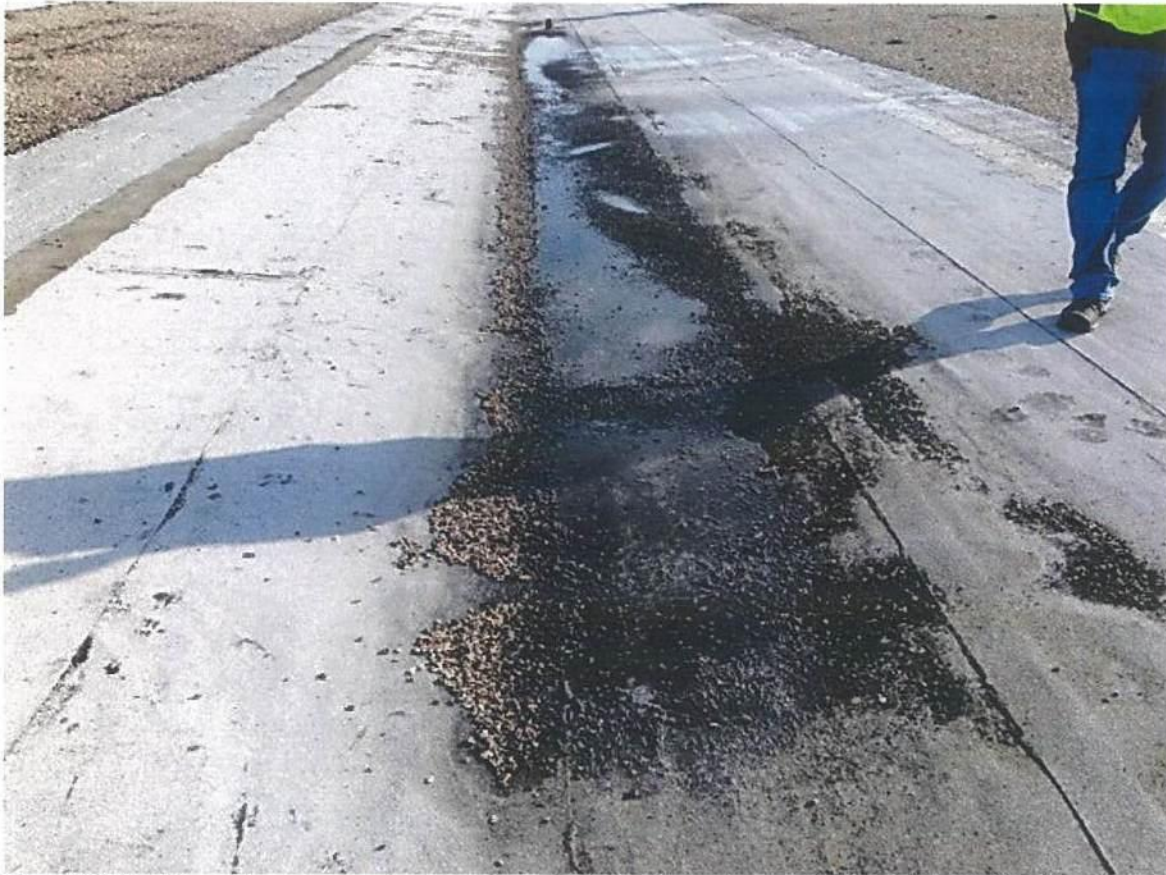
Photo #9760 View of ponding condensate water which has drained across the roof and ponding in valley near location #41 & 42 at the mineral surfaced modified bitumen roof patch at the west valley line of the Upper Roof north of expansion joint #9.
