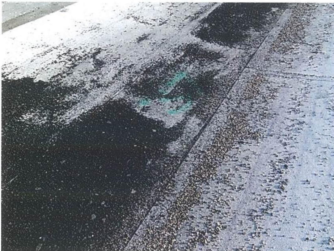
Photo #9753 View of entrapped moisture location #37 at the mineral surfaced modified bitumen roof patch at the east valley line of the Upper Roof north of expansion joint #8.
