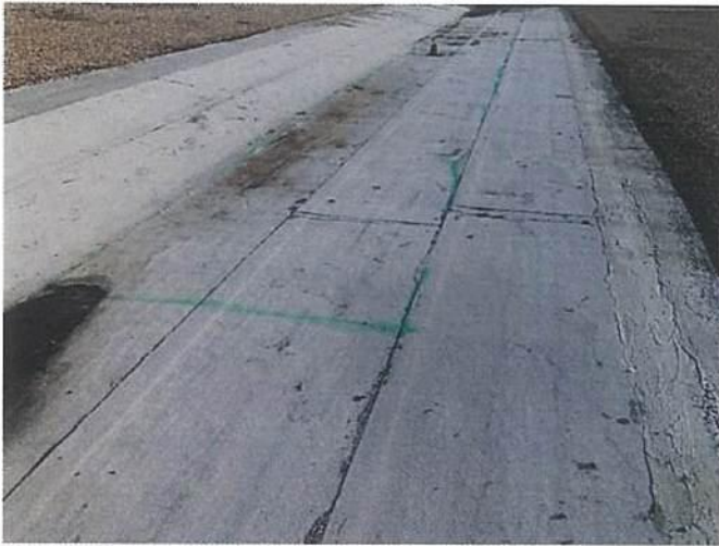
Photo #9746 View of entrapped moisture location #33 at the mineral surfaced modified bitumen roof patch at the west valley line of the Upper Roof south of expansion joint #8.
