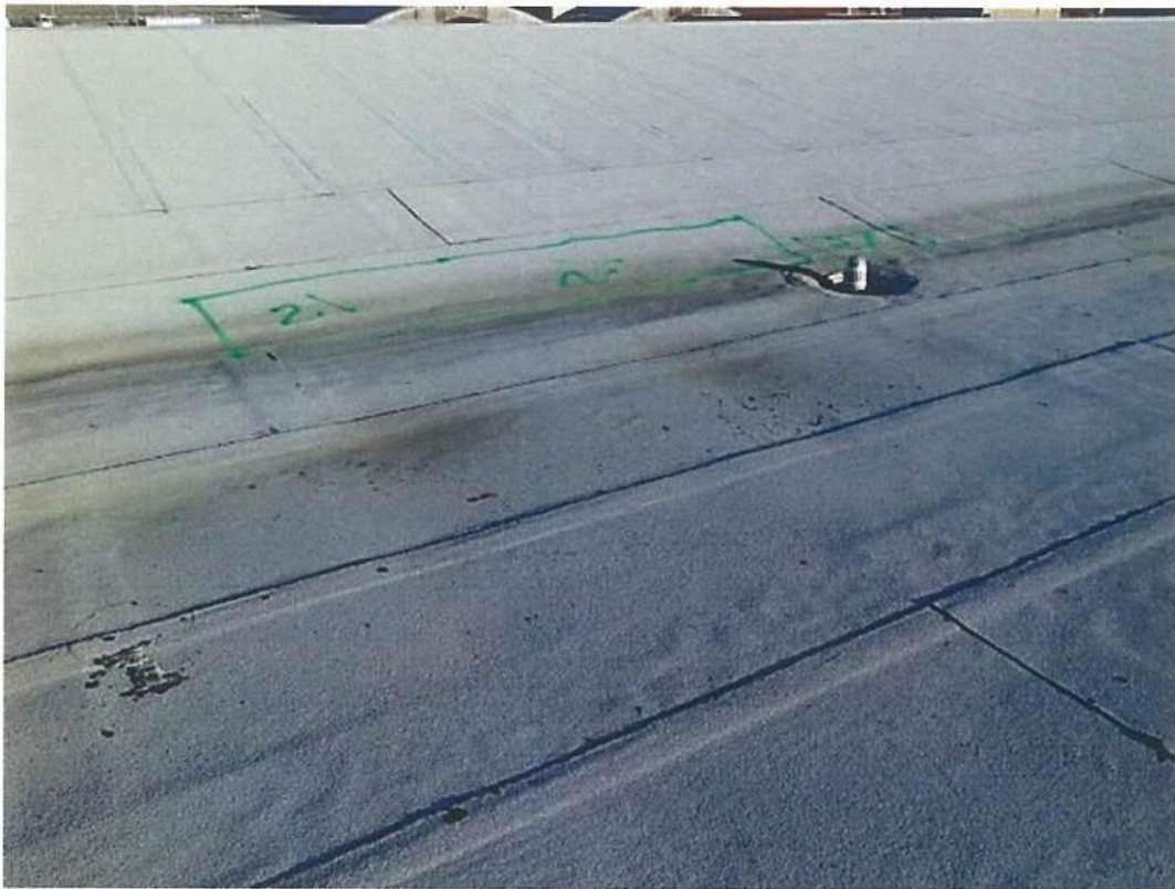
Photo #9707 View of entrapped moisture #21 near a roof drain at the west side of the Upper roof south of expansion joint #6.
