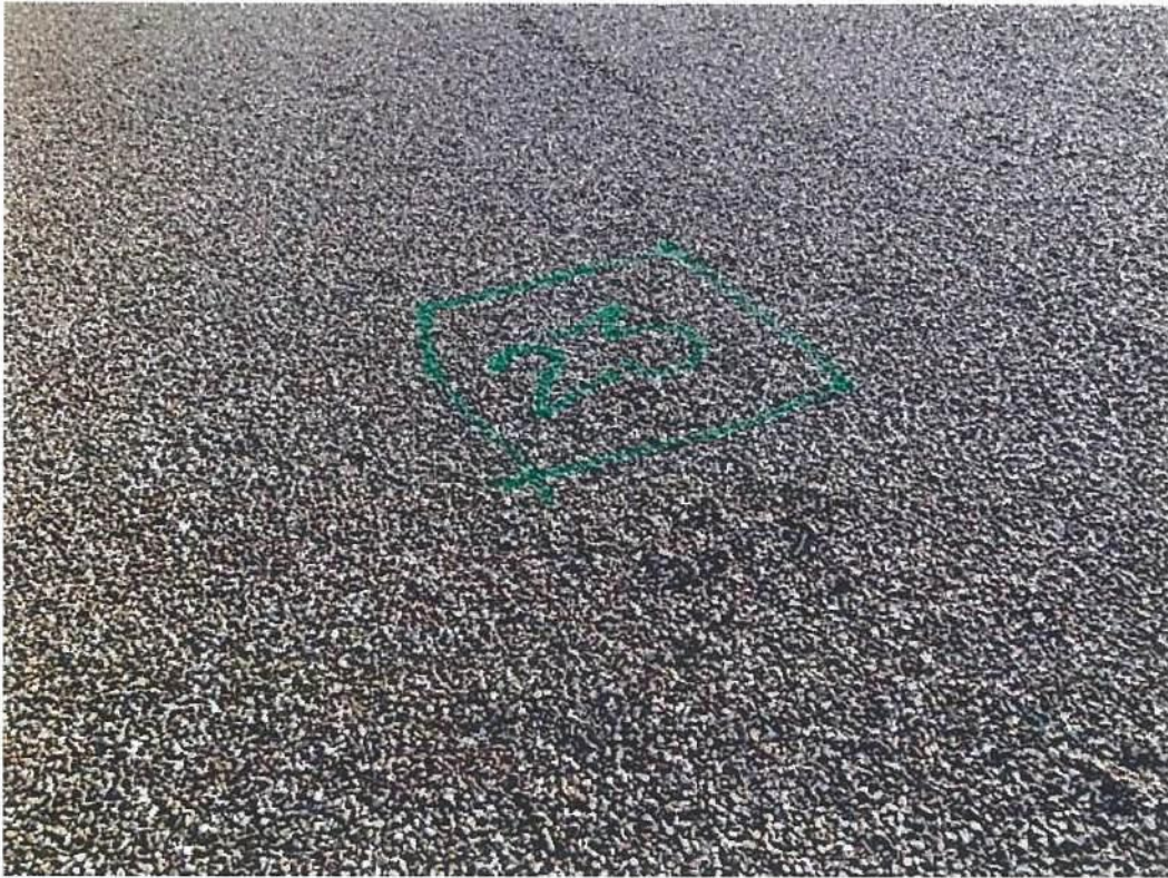
Photo #9716 View of entrapped moisture location #23 at the gravel surfaced built up roof area at the Upper roof north of expansion joint #6.
