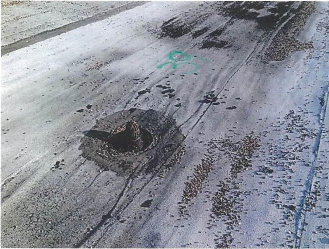
Photo #9755 View of entrapped moisture location #39 at the mineral surfaced modified bitumen roof patch at the east valley line of the Upper Roof north of expansion joint #8.
