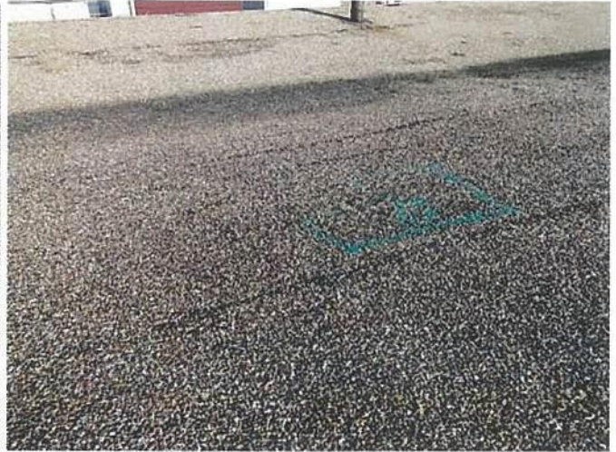
Photo #9715 View of entrapped moisture location #22 at the gravel surfaced built up roof area at the Upper roof north of expansion joint #6. Photo #9737 Entrapped moisture location #22
