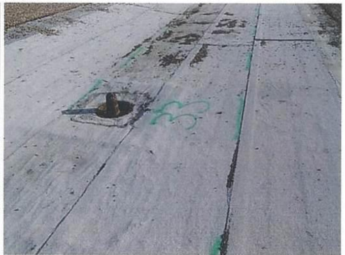
Photo #9747 View of entrapped moisture location #33 at the mineral surfaced modified bitumen roof patch at the west valley line of the Upper Roof south of expansion joint #8
