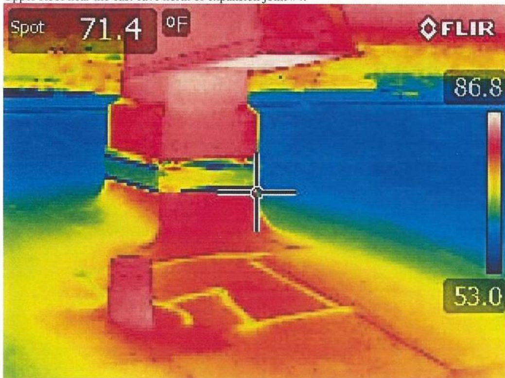
Photo #0462 View of area of entrapped moisture location #11 represented by red shaded area between plumbing vent and exhaust fan curb near the east eave of the Upper roof north of expansion joint #4.
