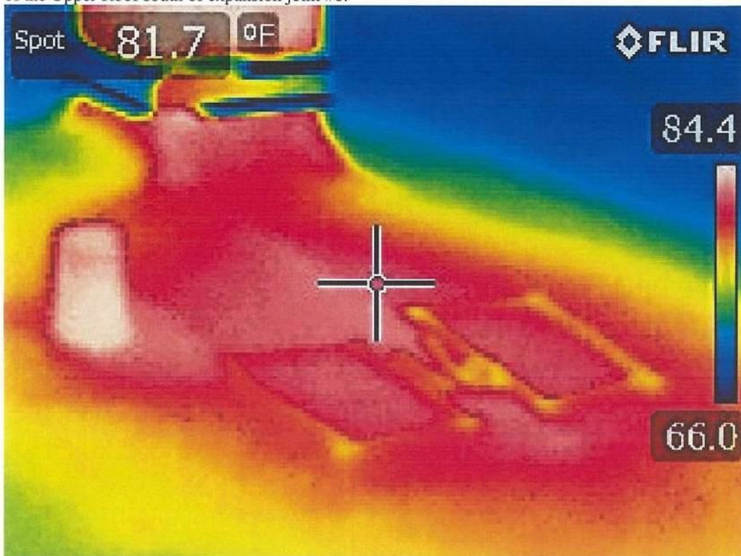
Photo #0472 View of entrapped moisture location #16 represented by red shaded area at the base of a plumbing vent and exhaust fan curb at the east side of the Upper Roof area south of expansion joint #6.
