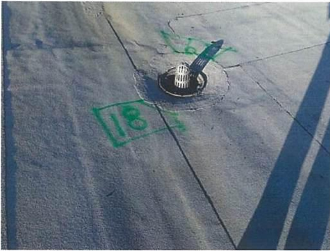
Photo #9704 View of entrapped moisture #18 near a roof drain Near the north side of the Upper Roof expansion joint #5. Photo #9705 View of entrapped moisture #19 at roof drain Near the north side of the Upper Roof expansion joint #5.
