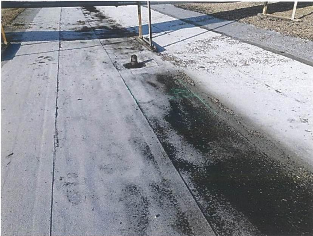
Photo #9763 View of entrapped moisture location #41 at the mineral surfaced modified bitumen roof patch at the west valley line of the Upper Roof north of expansion joint #8.
