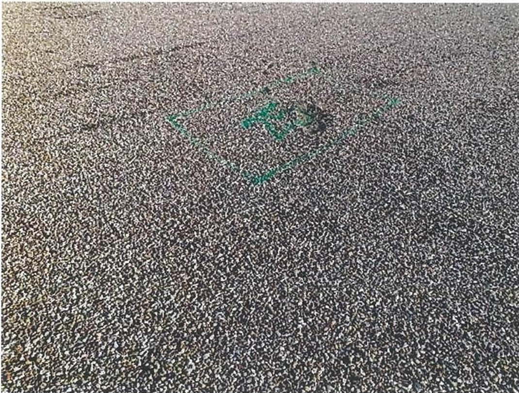
Photo #9714 View of entrapped moisture location #25 at the gravel surfaced built up roof area at the east side of the Upper roof north of expansion joint #6.
