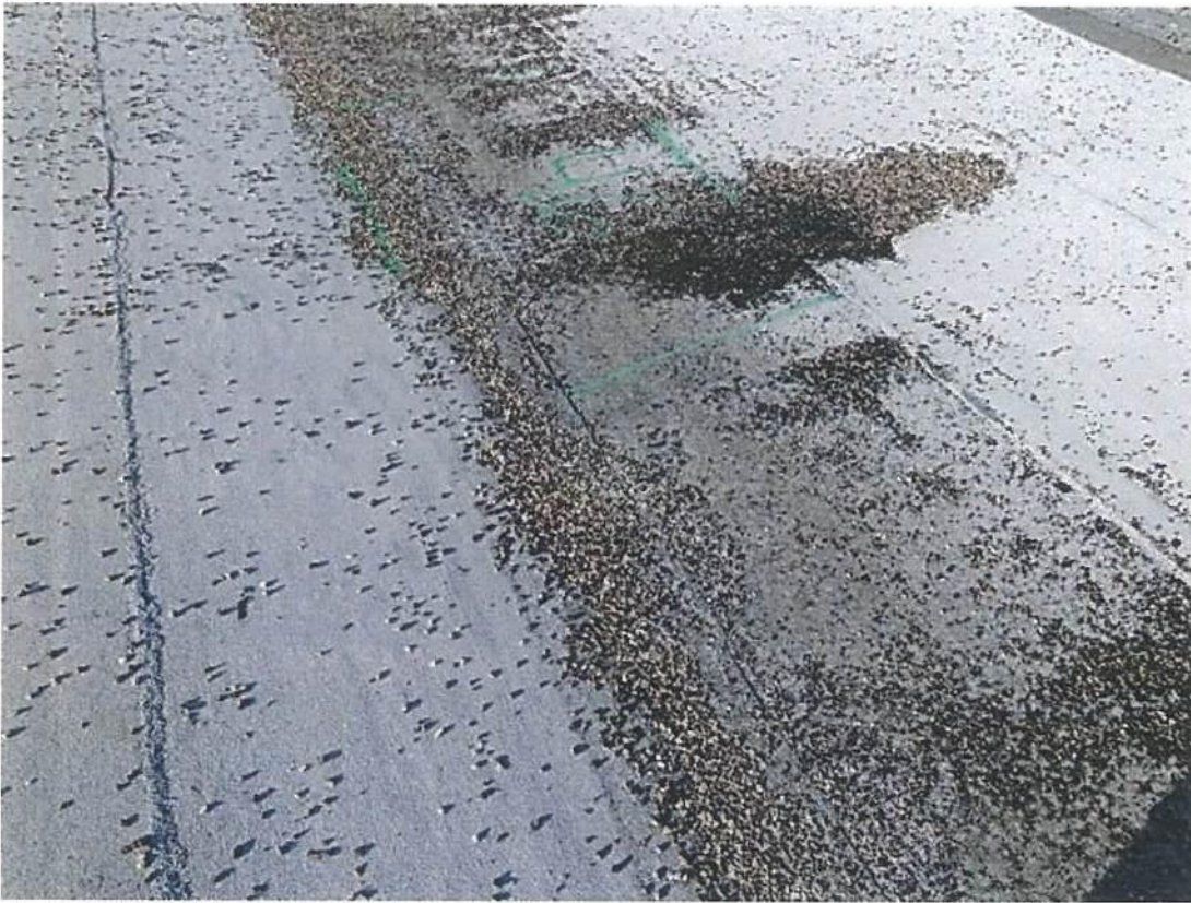
Photo #9770 View of area of entrapped moisture location #46 in east valley modified bitumen patch at the Upper Roof north of expansion joint #9.
