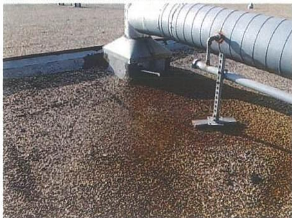
Photo #9764 Condensate draining on roof.
