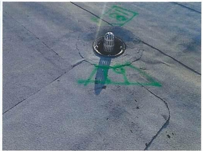
Photo #9704 View of entrapped moisture #18 near a roof drain Near the north side of the Upper Roof expansion joint #5. Photo #9705 View of entrapped moisture #19 at roof drain Near the north side of the Upper Roof expansion joint #5.
