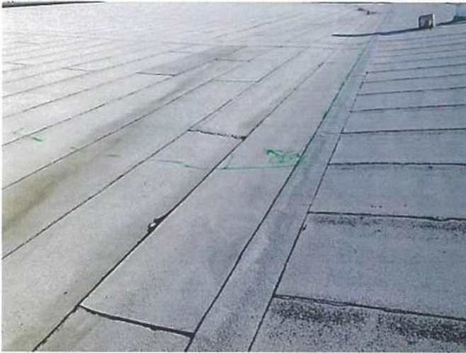
Photo #9772 View of entrapped moisture location #50 at the Upper Roof near the east valley north of expansion joint #11.
