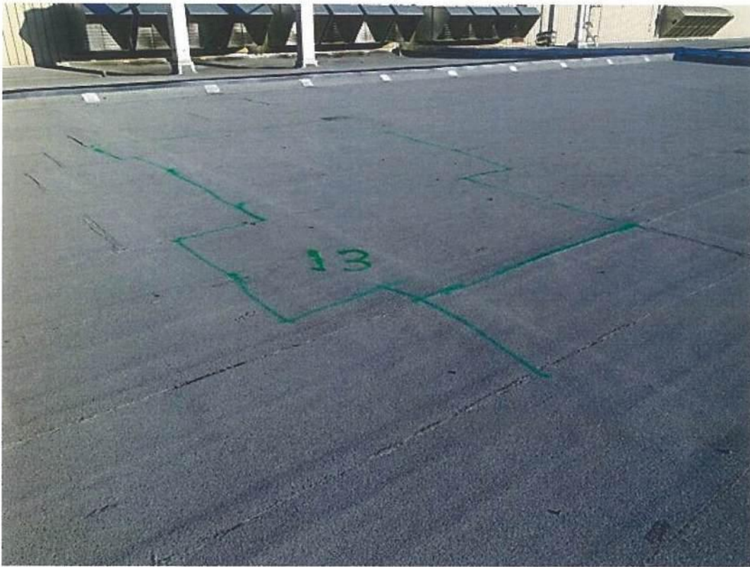
Photo #9710 View of entrapped moisture location #13 at the east 1/2 of the Lower Roof south of Expansion joint #6.
