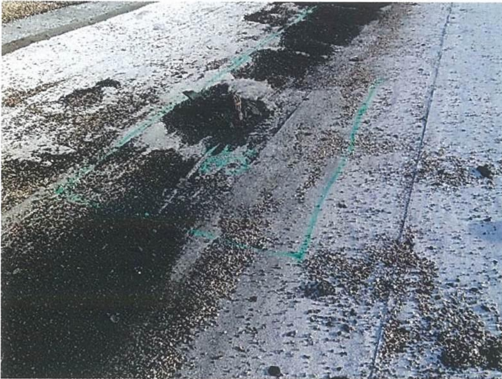
Photo #9751 View of entrapped moisture location #35 at the mineral surfaced modified bitumen roof patch at the east valley line of the Upper Roof north of expansion joint #8.
