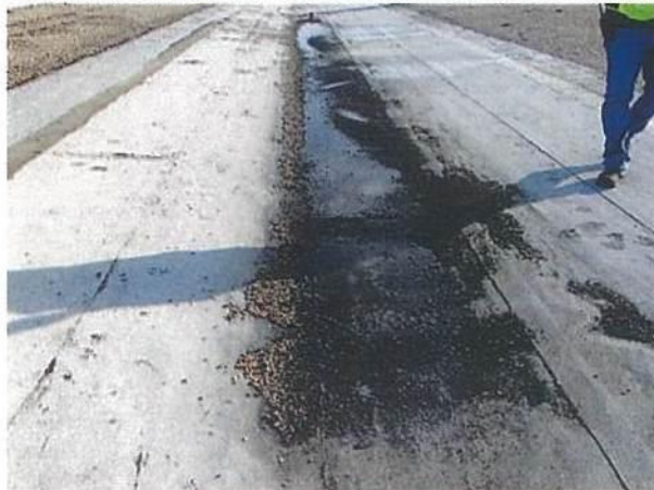
Photo #9760 Ponding in valley line caused by Condensate allowed to drain on roof.
