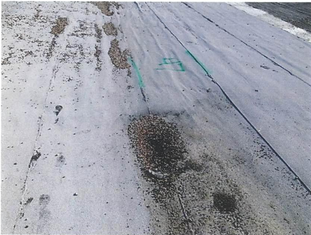
Photo #9768 View of area of entrapped moisture location #47 in west valley modified bitumen patch at the Upper Roof south of expansion joint #10.
