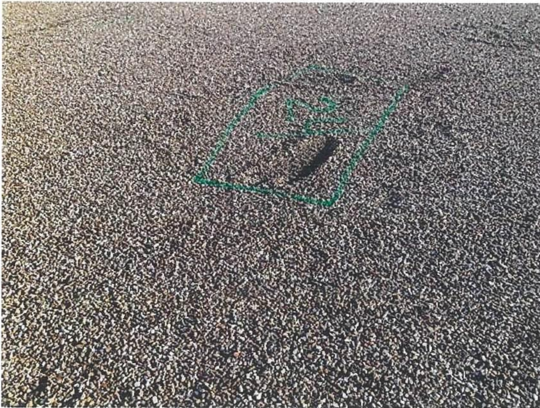
Photo #9713 View of entrapped moisture location #24 at the gravel surfaced Upper Roof north of expansion joint #6.
