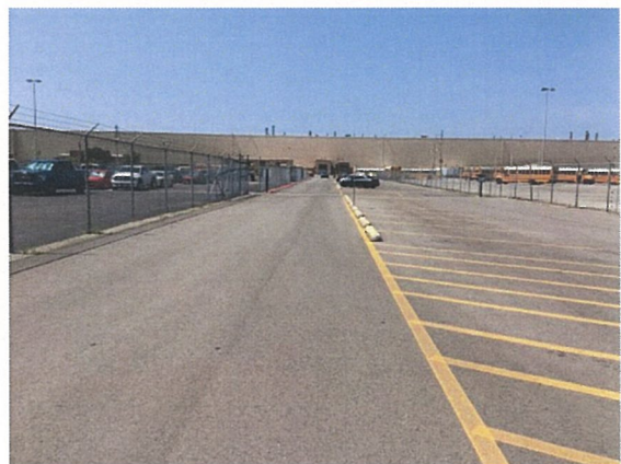
Area 1 South Driveway (N Mingo Rd) – Concrete (End of Driveway new Asphalt Pavement)
