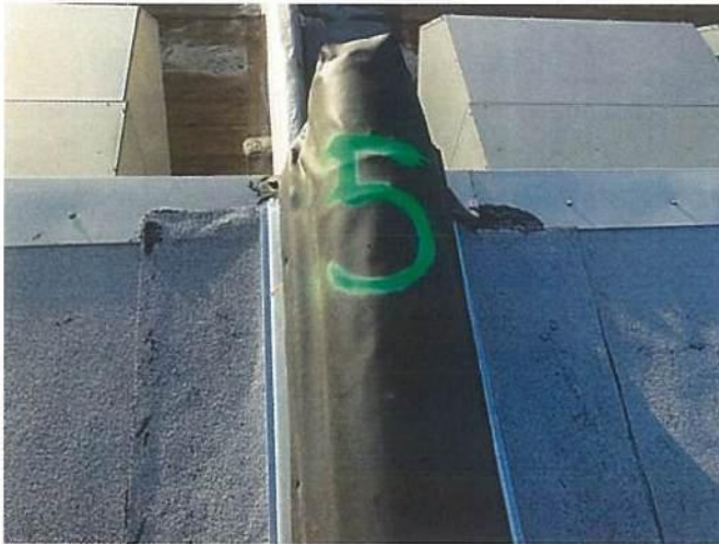
Photo #9703 View of Upper roof expansion joint #5.
