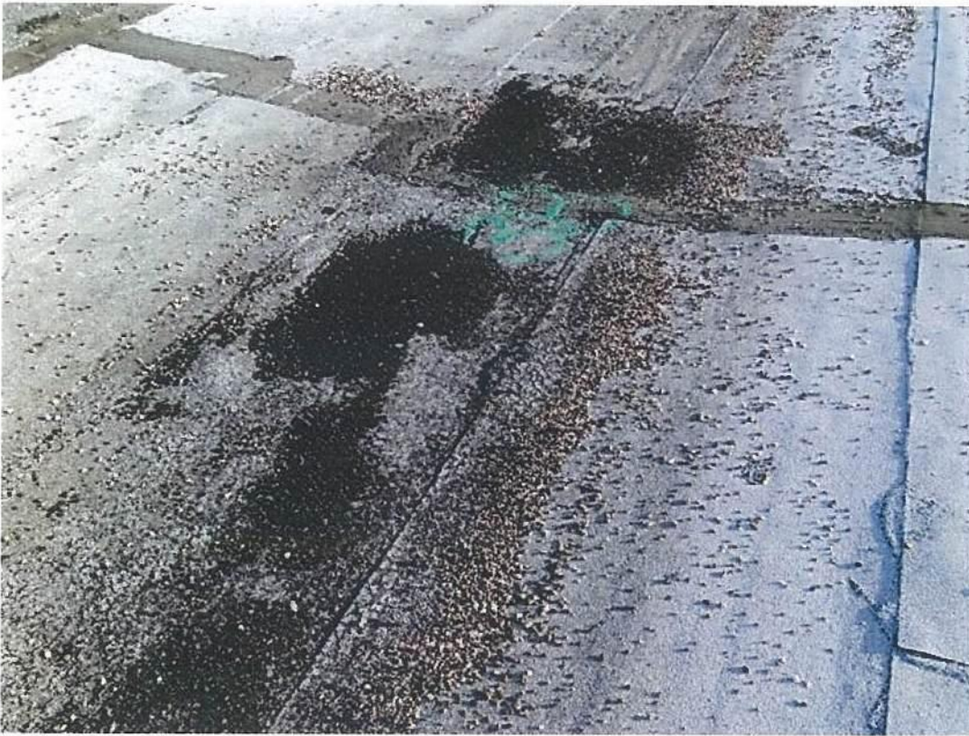
Photo #9754 View of entrapped moisture location #38 at the mineral surfaced modified bitumen roof patch at the east valley line of the Upper Roof north of expansion joint #8.
