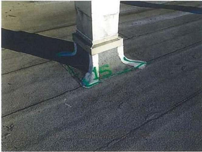
Photo #9712 View of entrapped moisture location #15 at base of a flue stack at the Lower roof south of expansion joint #6. Photo #9725 View of missing weather hood at flue stack at Entrapped moisture location #15.
