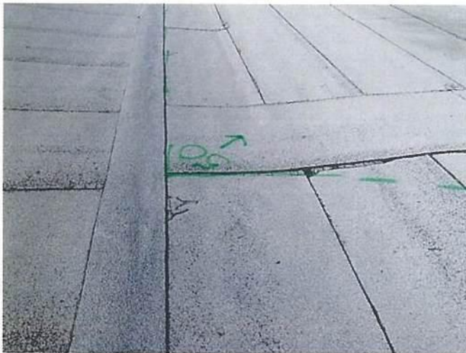
Photo #9775 View of entrapped moisture location #50 at the Upper Roof near the east valley north of expansion joint #11.
