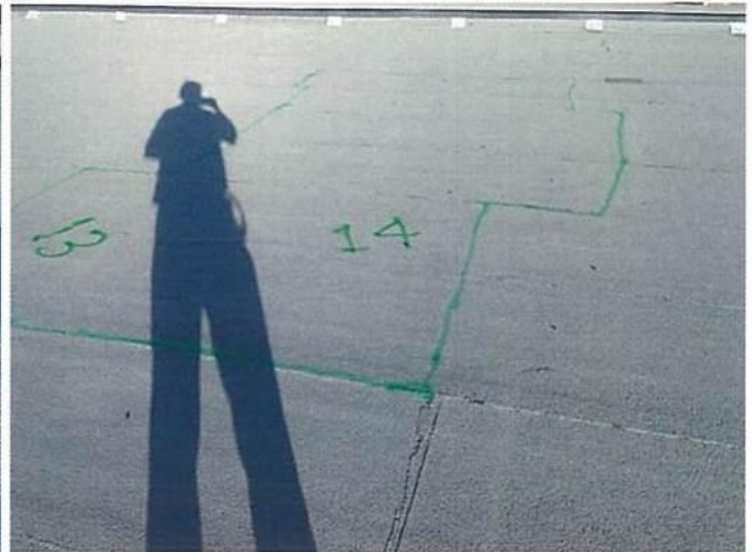
Photo #9711 View of large area of entrapped moisture #14 South of expansion joint #6 at the Lower East roof.
