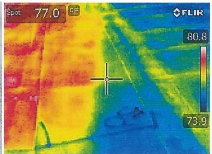
Photo #0550 View of entrapped moisture location #50 at the Upper Roof near the east valley north of expansion joint #11.
