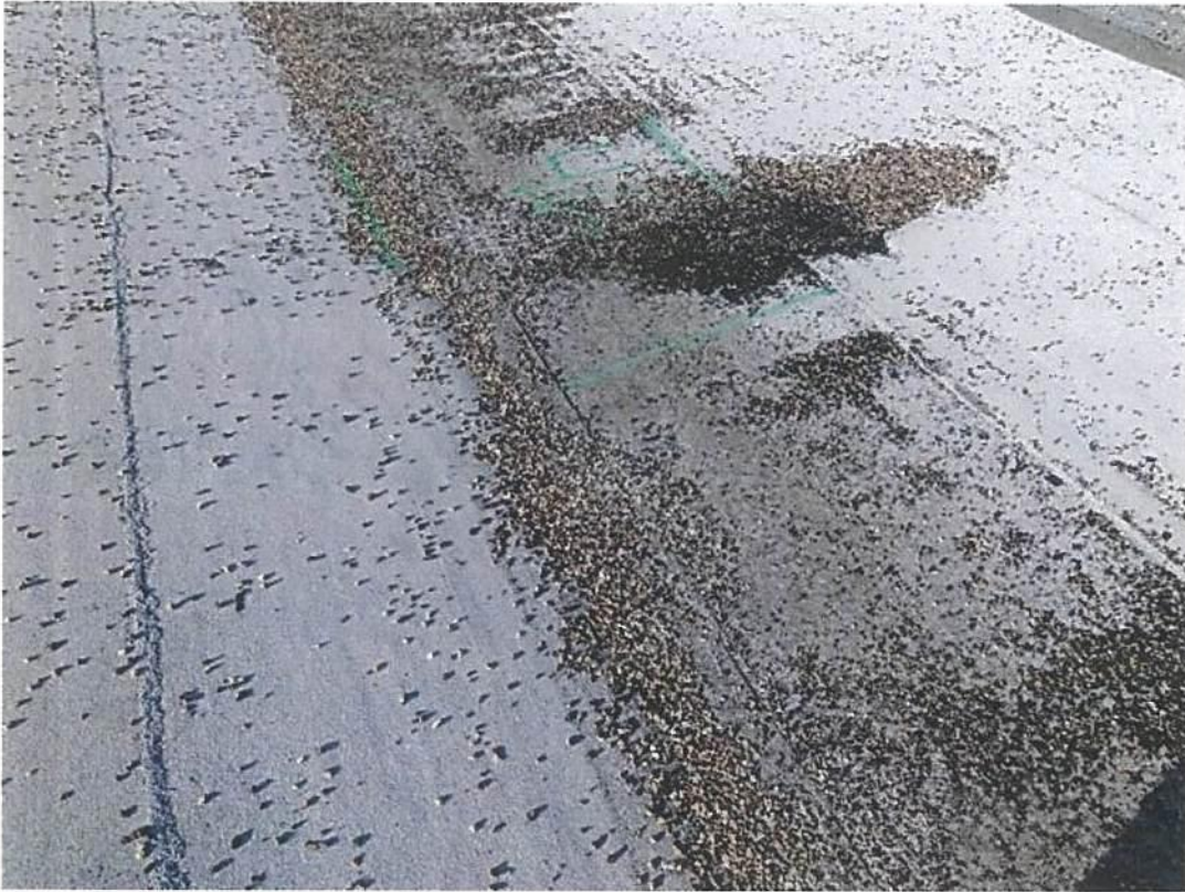
Photo #9770 View of area of entrapped moisture location #49 in west valley modified bitumen patch at the Upper Roof north of expansion joint #9.
