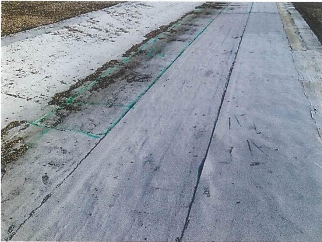
Photo #9742 View of entrapped moisture location #29 at the mineral surfaced modified bitumen roof patch at the west valley line of the Upper Roof north of expansion joint #7.
