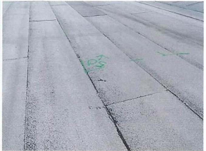
Photo #9773 View of entrapped moisture location #50 at the Upper Roof near the east valley north of expansion joint #11.
