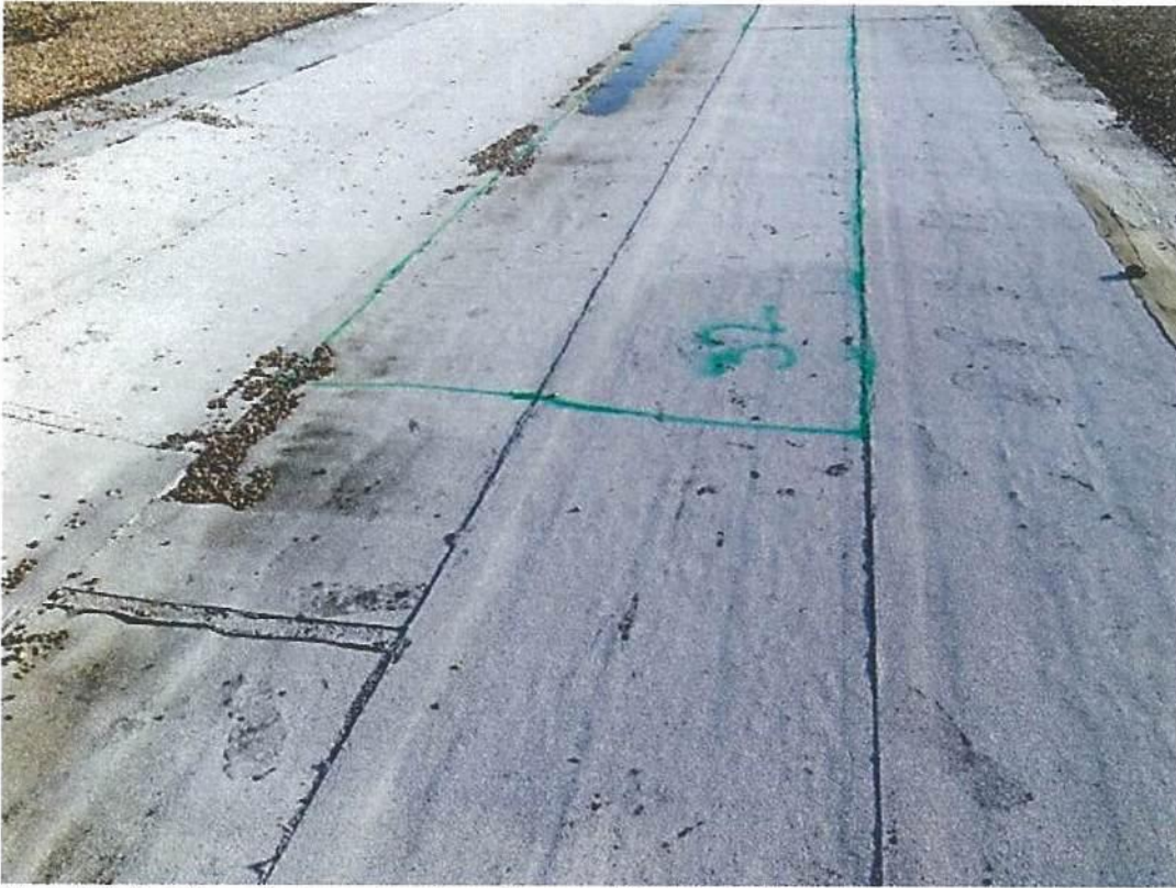
Photo #9745 View of entrapped moisture location #32 at the mineral surfaced modified bitumen roof patch at the east valley line of the Upper Roof south of expansion joint #8.
