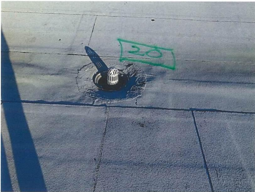
Photo #9706 View of entrapped moisture location #20 near a roof drain at the west side of the Upper roof north of expansion joint #5.
