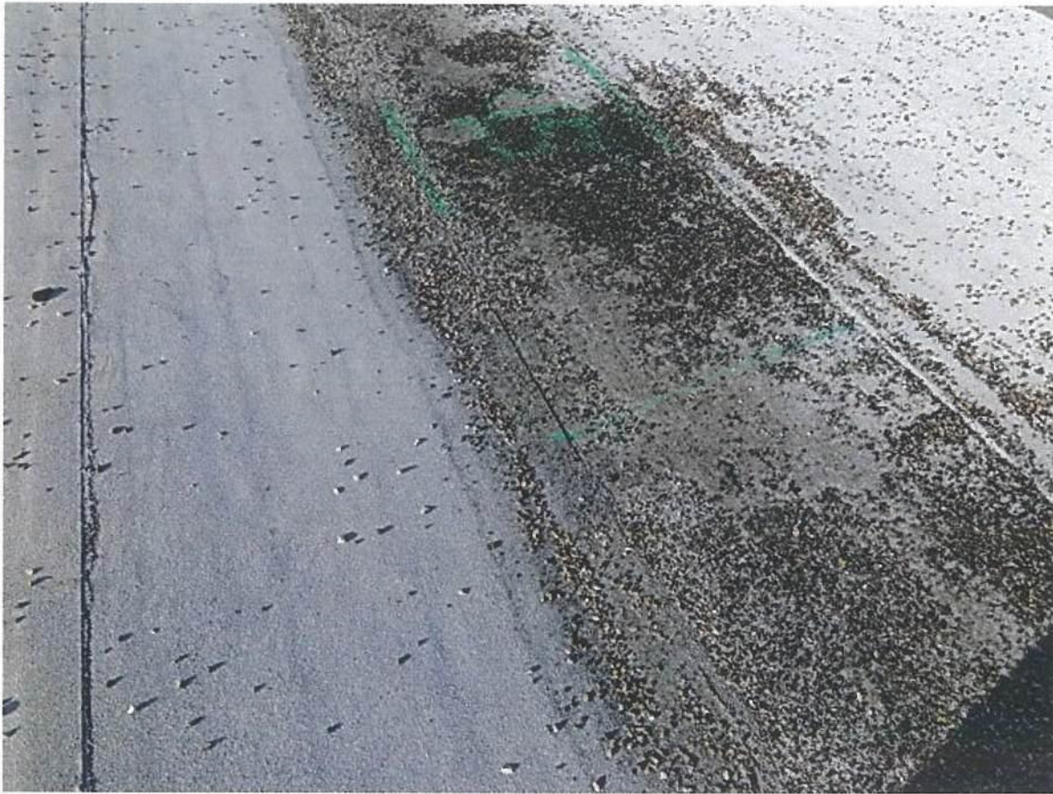
Photo #9769 View of area of entrapped moisture location #45 in east valley modified bitumen patch at the Upper Roof north of expansion joint #9.
