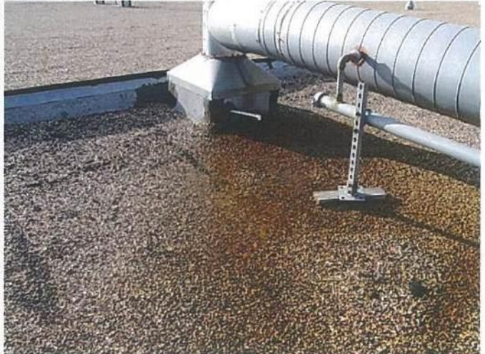
Photo #9764 Condensate water piped through curb at Duct roof penetration. Water drains across the roof causing roof membrane rotting and leaks at location #41.
