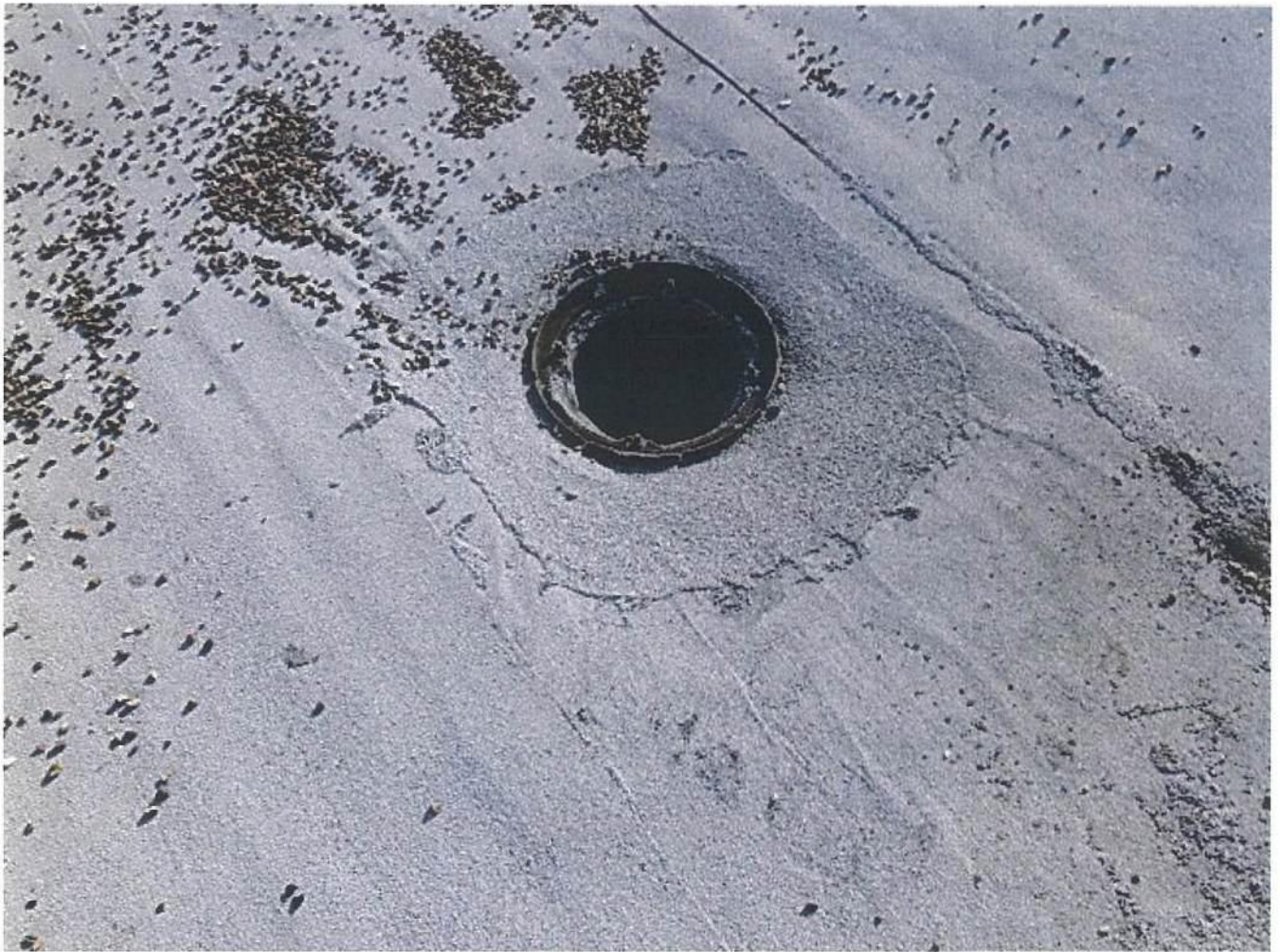
Photo #9771 View of roof drain missing strainer basket at the east valley modified bitumen at the Upper Roof south of expansion joint #10.
