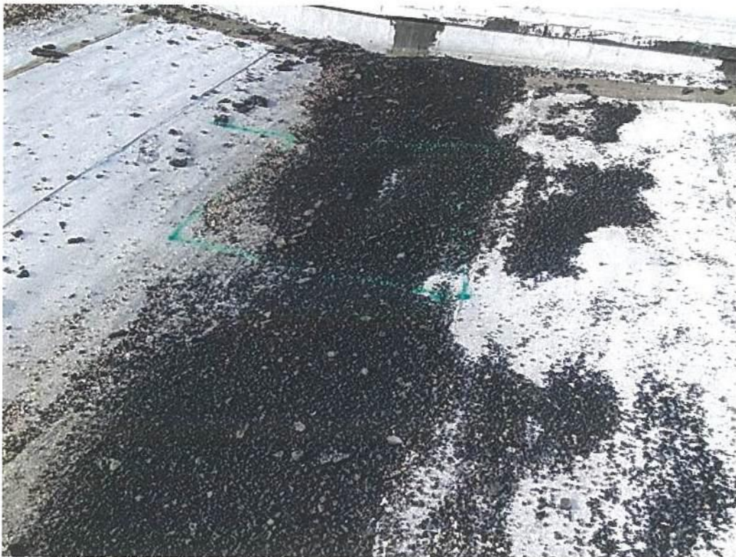
Photo #9750 View of entrapped moisture location #34 at the mineral surfaced modified bitumen roof patch at the east valley line of the Upper Roof north of expansion joint #8.
