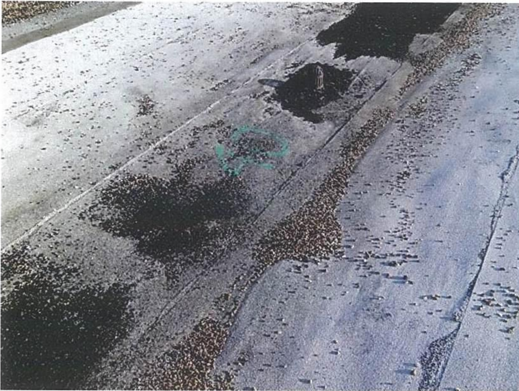
Photo #9756 View of entrapped moisture location #40 at the mineral surfaced modified bitumen roof patch at the east valley line of the Upper Roof south of expansion joint #9.
