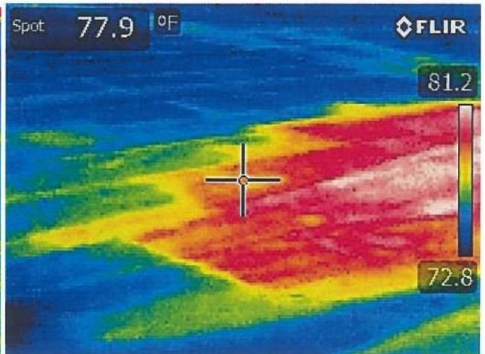
Photo #0554 View of entrapped moisture location #50 at the Upper Roof near the east valley north of expansion joint #11.
