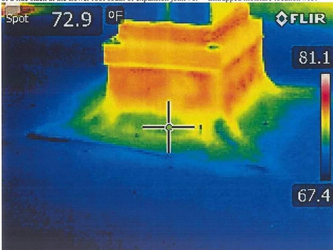
Photo #0470 View of entrapped moisture location #15 represented by red, yellow and green shaded areas at the base of a flue curb at the west 1/2 of the Lower Roof area south of expansion joint #6.
