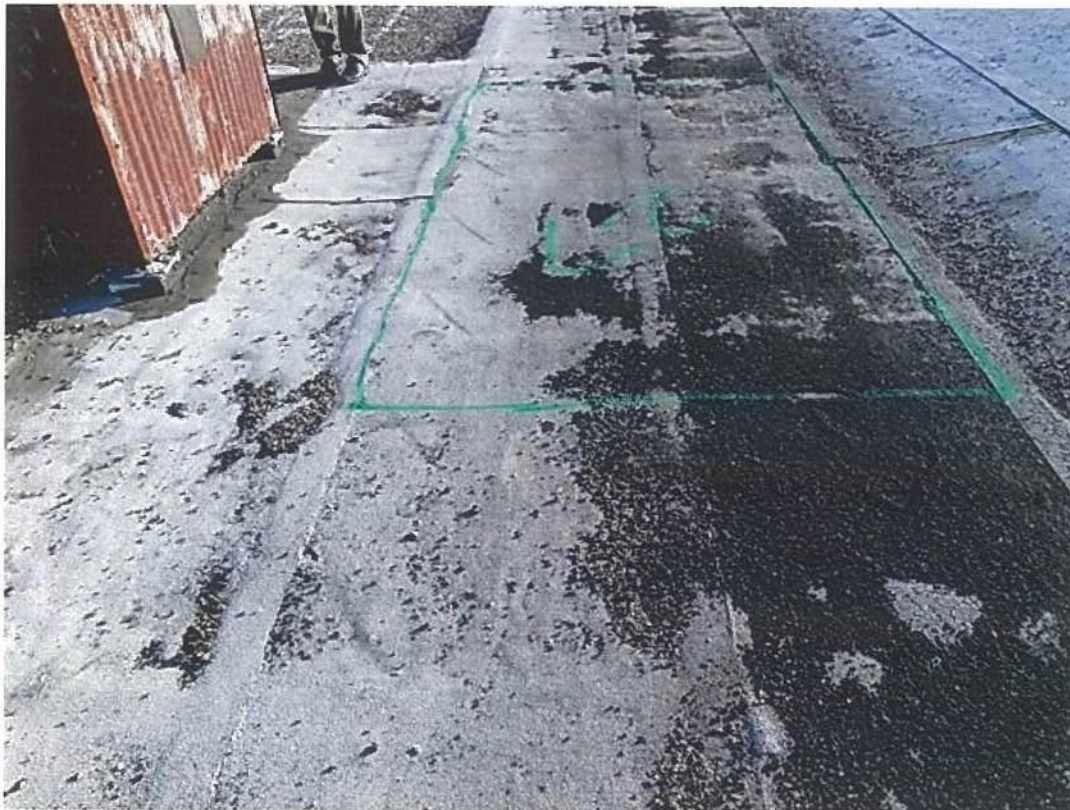
Photo #9717 View of entrapped moisture location #27 at the mineral surfaced modified bitumen patched roof area at the Upper roof east valley north of expansion joint #7.
