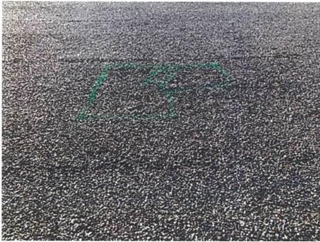
Photo #9715 View of entrapped moisture location #22 at the gravel surfaced built up roof area at the Upper roof north of expansion joint #6. Photo #9737 Entrapped moisture location #22
