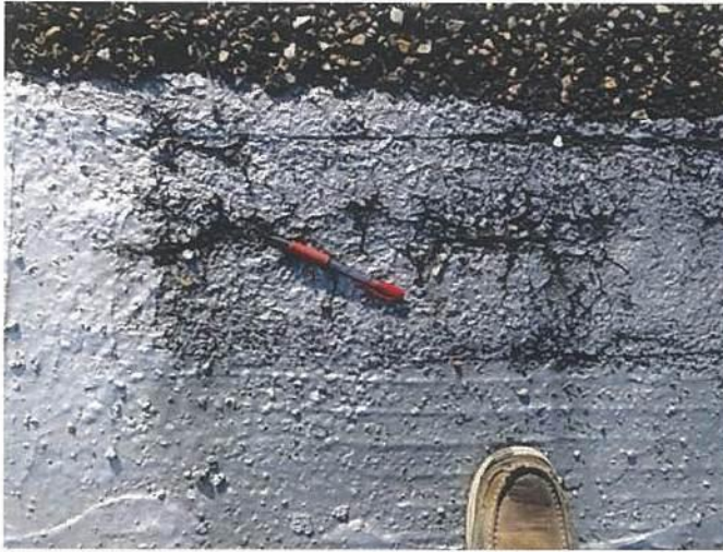
Photo #9767 View of split and deteriorated built-up roof membrane near area of entrapped moisture location #42.
