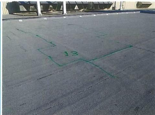
Photo #9710 Entrapped moisture Location #13. Size 12'x20'.
