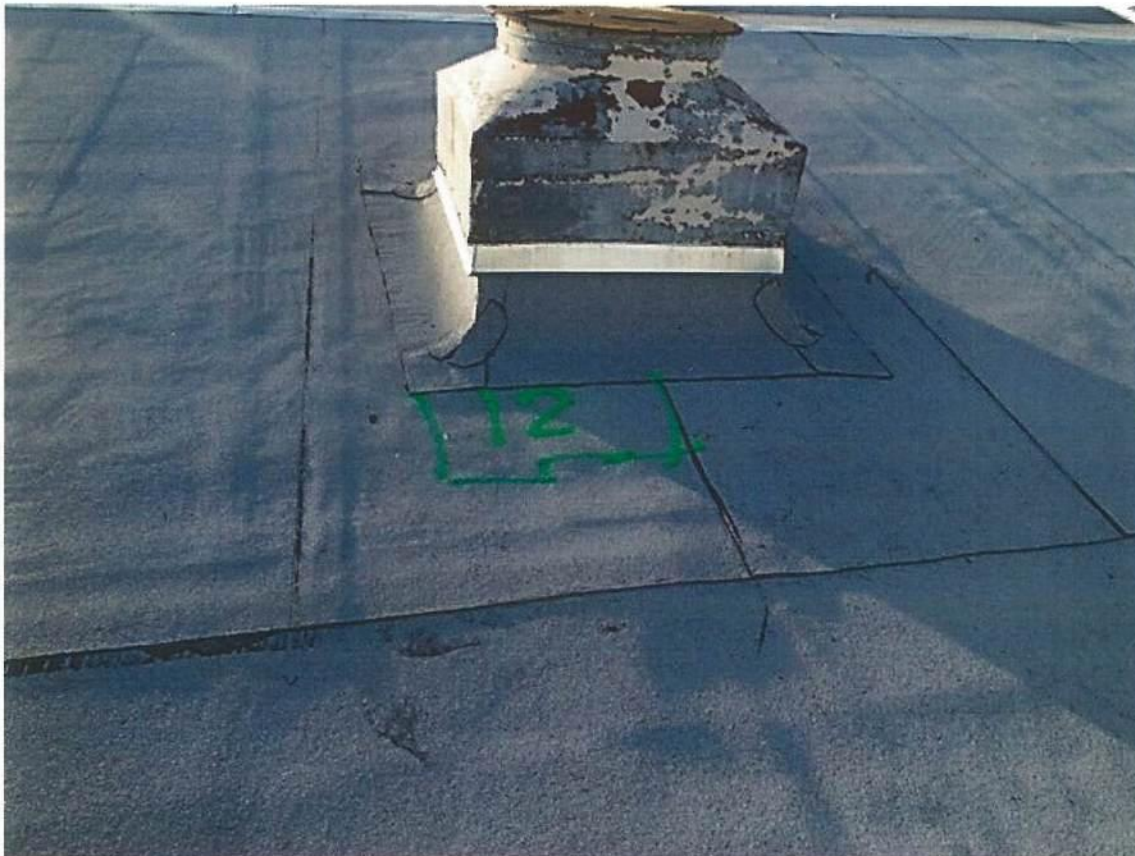
Photo #9701 View of entrapped moisture #12 at the base of an abandoned exhaust fan curb near the east eave of the Upper Roof north of Expansion joint #4.
