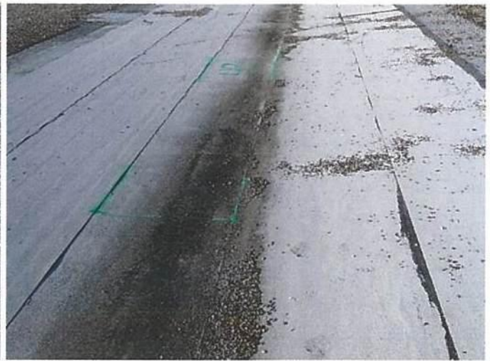
Photo #9765 View of entrapped moisture location #42 in the west valley at the Upper Roof north of expansion joint 8.
