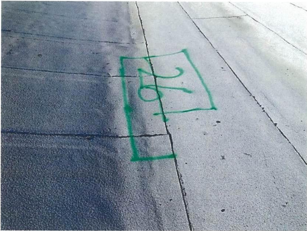
Photo #9718 View of entrapped moisture location #26 at the mineral surfaced modified bitumen roof at the east valley line of the Lower Roof north of expansion joint #7.
