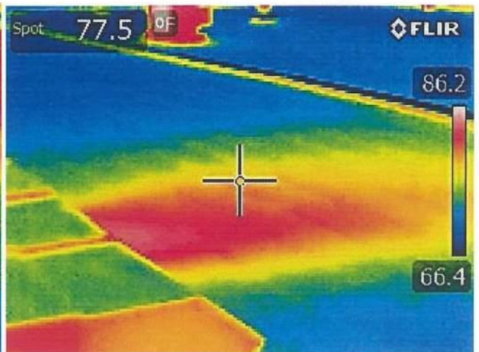
Photo #0544 View of heat from air blown out of exhaust fans in the offset wall at the Lower Roof north of expansion joint 10 as seen from the east eave of the Upper Roof.
