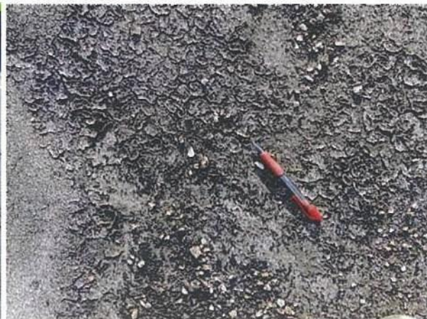
Photo #9761 Delaminated capsheet due to long term exposure to ponding condensate water.
