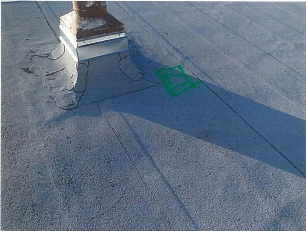
Photo #9709 View of entrapped moisture location 17 near base of an exhaust fan curb at the east side of the Upper Roof south of expansion joint #6.
