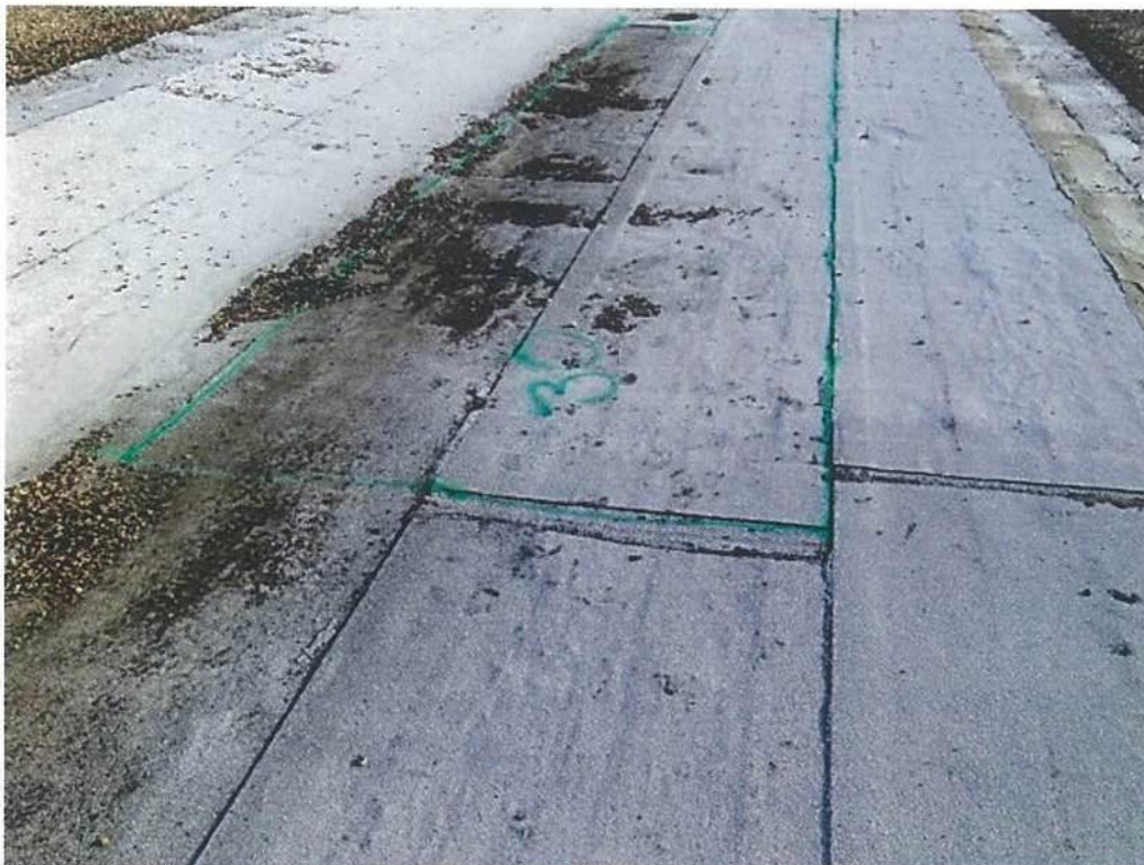
Photo #9743 View of entrapped moisture location #30 at the mineral surfaced modified bitumen roof patch at the west valley line of the Upper Roof south of expansion joint #8.
