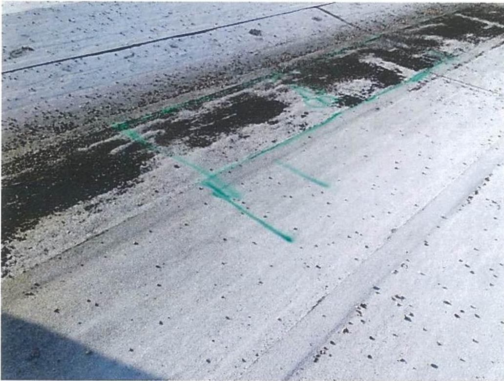
Photo #9749 View of entrapped moisture location #28 at the mineral surfaced modified bitumen roof patch at the east valley line of the Upper Roof south of expansion joint #8.
