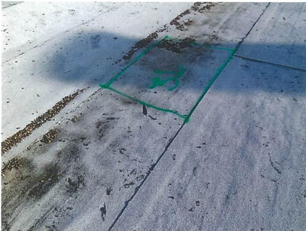
Photo #9744 View of entrapped moisture location #31 at the mineral surfaced modified bitumen roof patch at the west valley line of the Upper Roof south of expansion joint #8.
