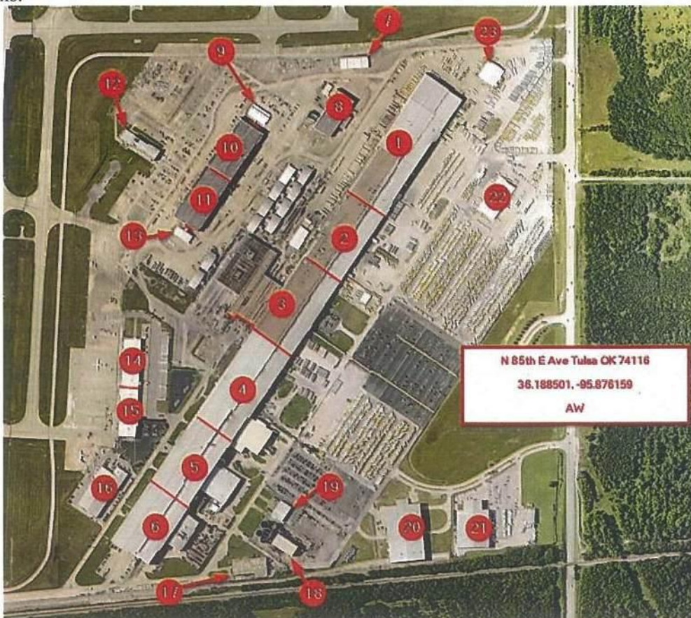
Aerial View of Roof. Navistar IC Bus, LLC Plant is in Sections 1,2,3 & 4 of the B001 Bldg.
