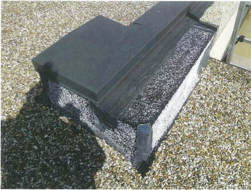
Photo #13 View of Roof Area 3 parapet coping.
