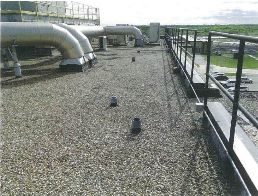
Photo #10 View of the south side of Roof Area 1 looking east.
