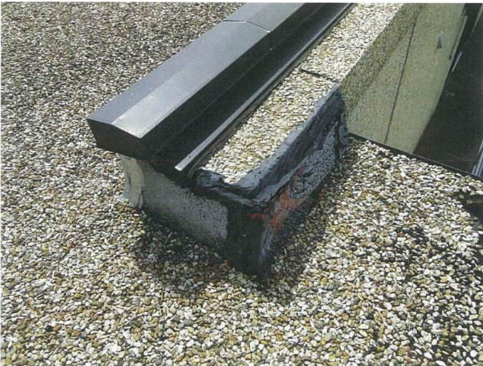
Photo #6 View of the existing aggregate concrete parapet wall and existing metal coping at the Filter Gallery Roof.
