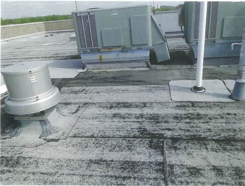
Photo #7 View of exhaust fan and HVAC unit curbs.
