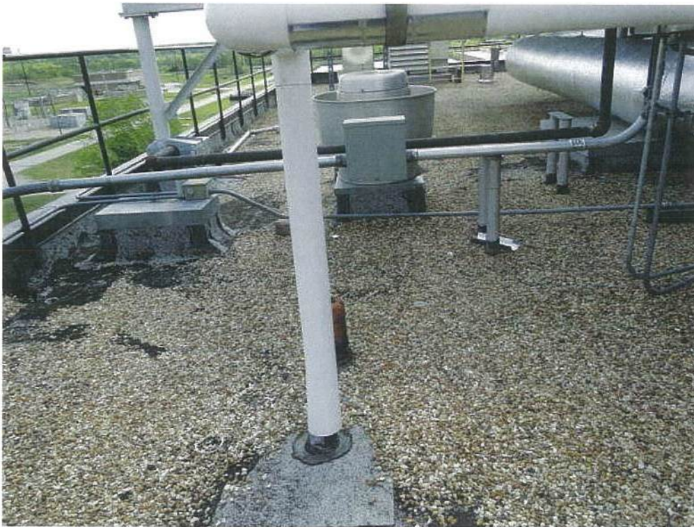
Photo #4 View of piping & equipment platform supports to remain at north side of Roof Area 1.
