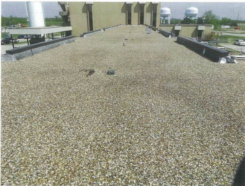
Photo #1 View of Filter Gallery Roof looking north.
