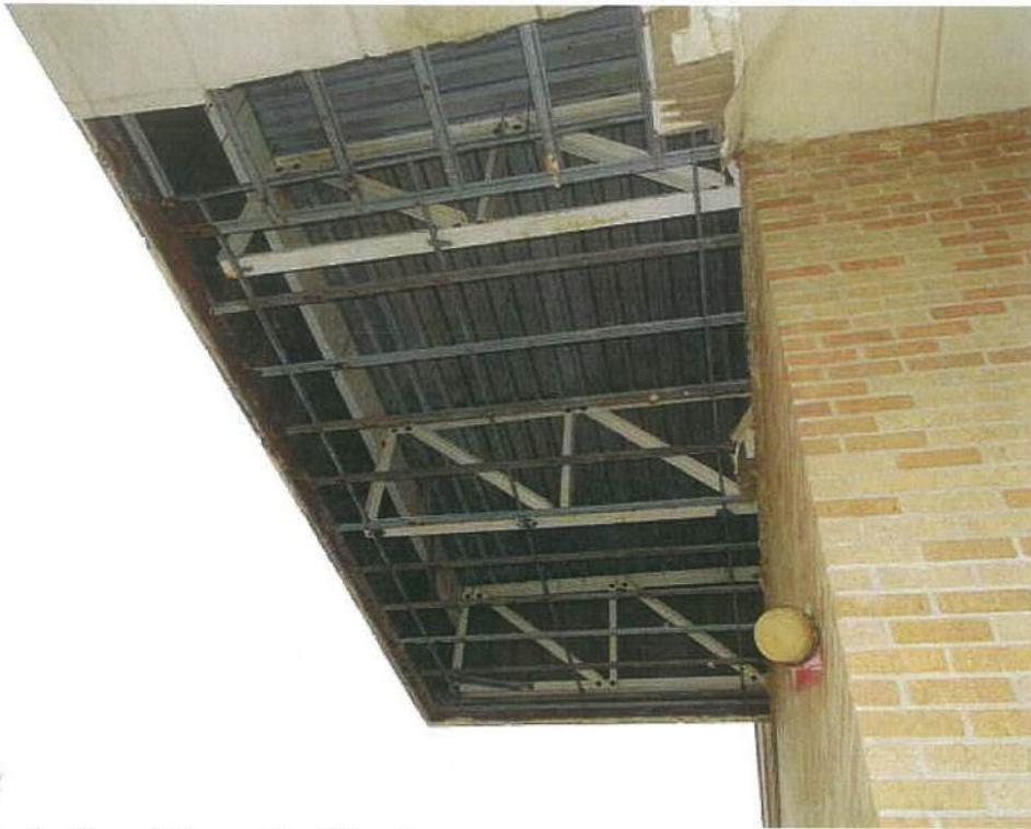
Photo #1 View of Canopy Roof Structure.
