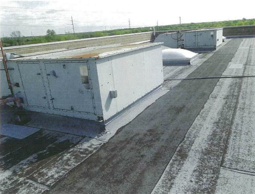
Photo #8 View of roof top mechanical equipment and curb mounted skylight.
