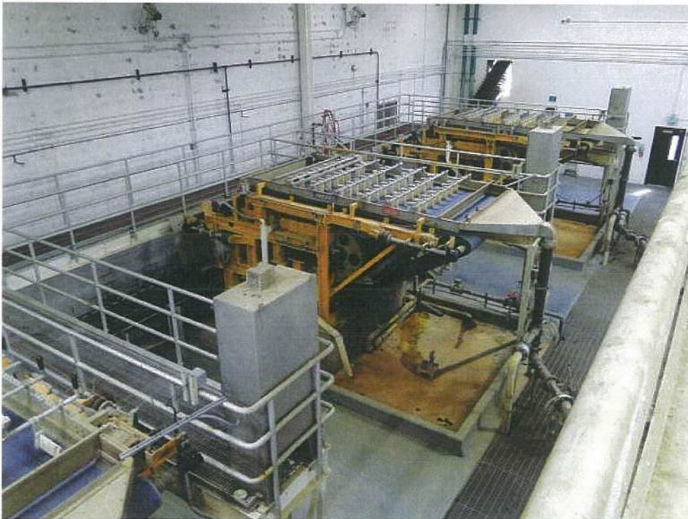
Photo #4 View of interior machinery to be protected from falling debris during roof demolition.
