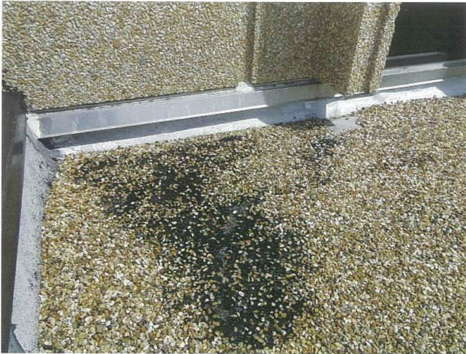
Photo #5 View of existing metal counter flashing to remain at the Filter Gallery Roof offset wall at the south side of the Administration Building.
