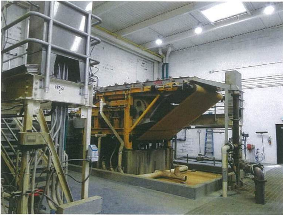
Photo #3 View of steel deck roof structure and interior machinery to be protected from falling debris during roof demolition.
