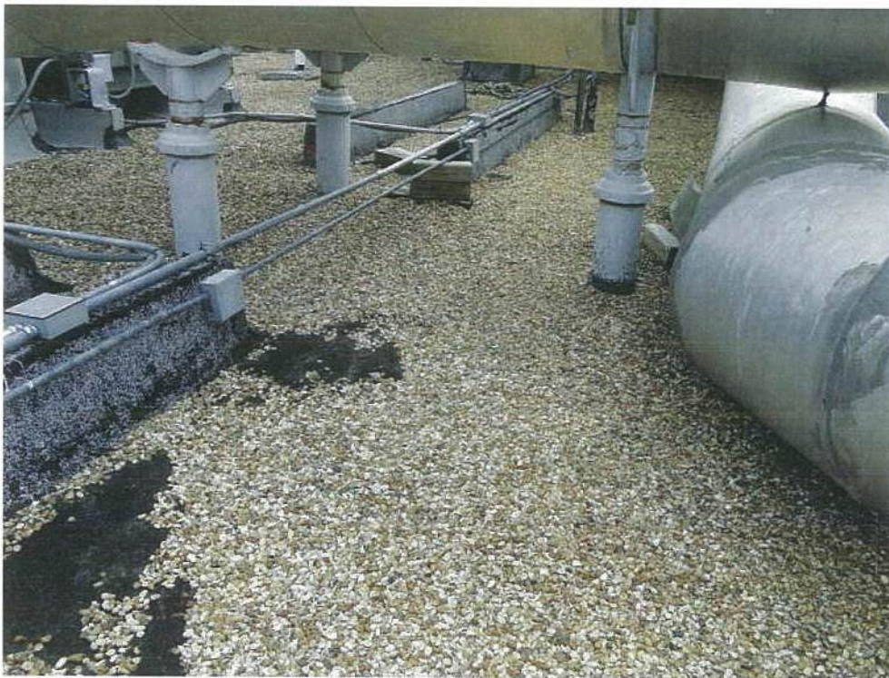
Photo #2 View of duct & equipment support curbs to be removed. Duct to be relocated by others.
