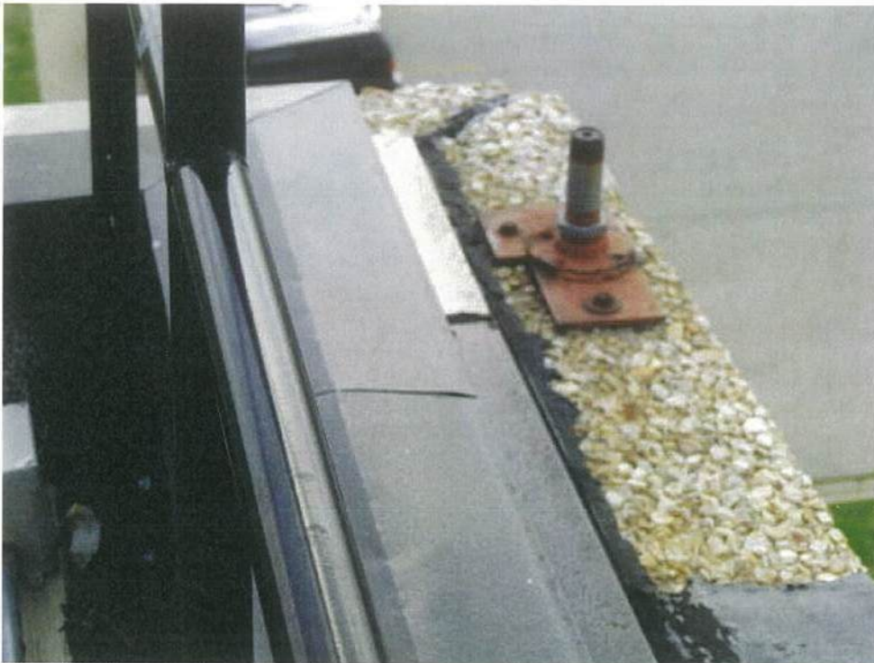
Photo #9 View of existing security camera mounting bracket to be removed at southeast corner of the Roof Area 1 parapet wall.
