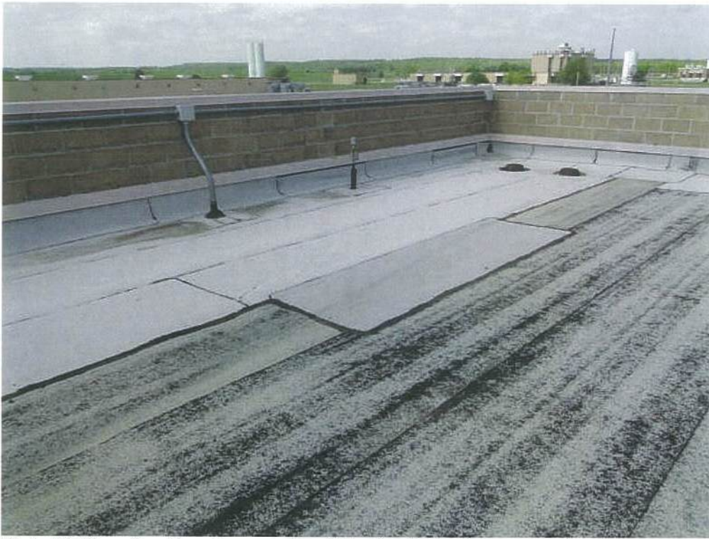
Photo #5 View of southwest corner of roof showing drains & parapet wall.
