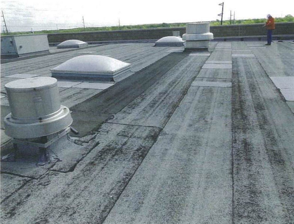
Photo #6 View of center of roof showing exhaust fans and skylights.
