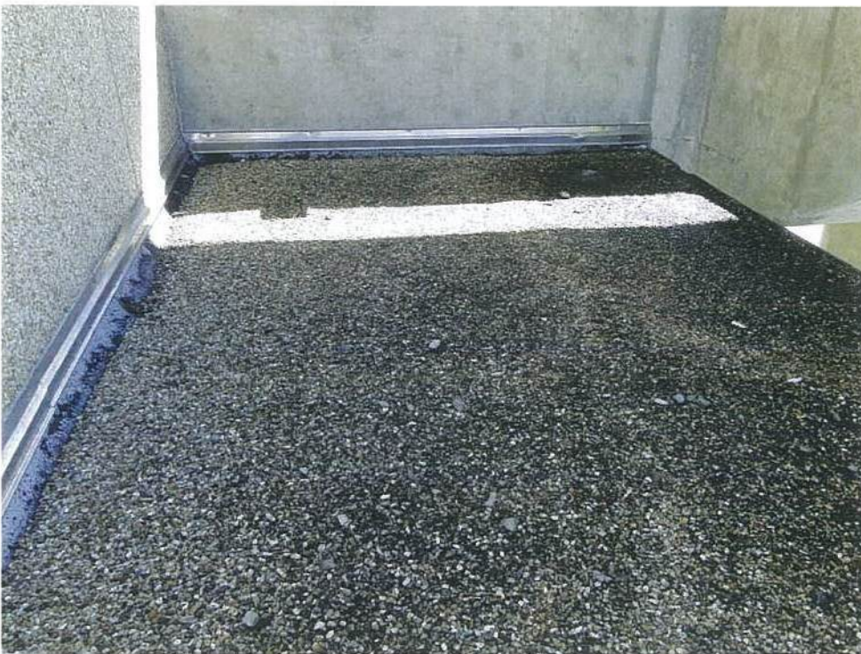
Photo #4 View of Existing Canopy Roof looking north.
