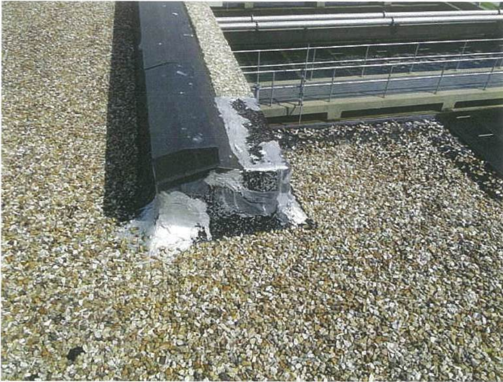
Photo #3 View of Filter Gallery Roof parapet wall & existing metal coping.
