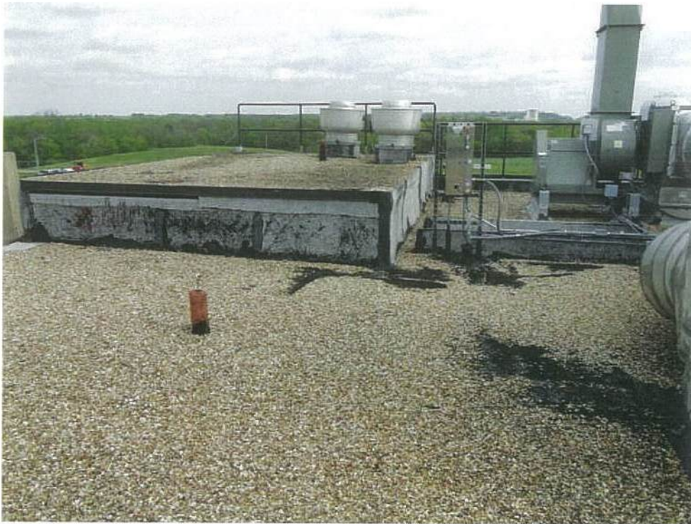
Photo #1 View of Elevator Penthouse Roof Area 2.
