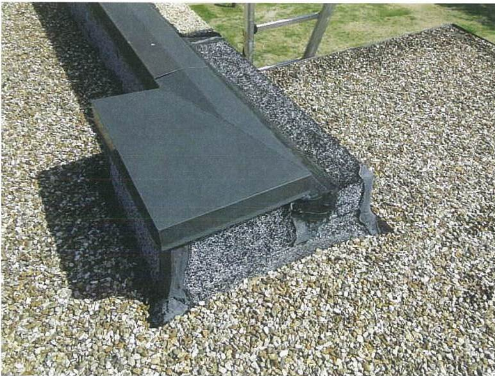
Photo #12 View of parapet wall coping at Roof Area 3 east side.
