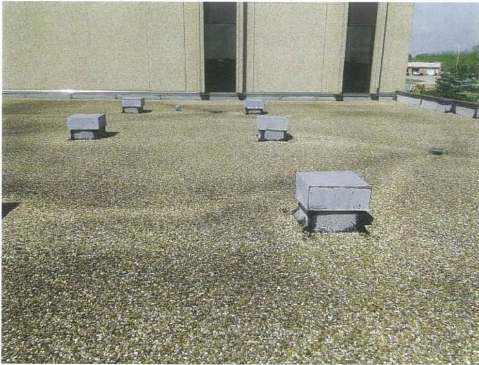
Photo #11 View of Roof Area 3 looking west. Future column stub-ups are to remain.
