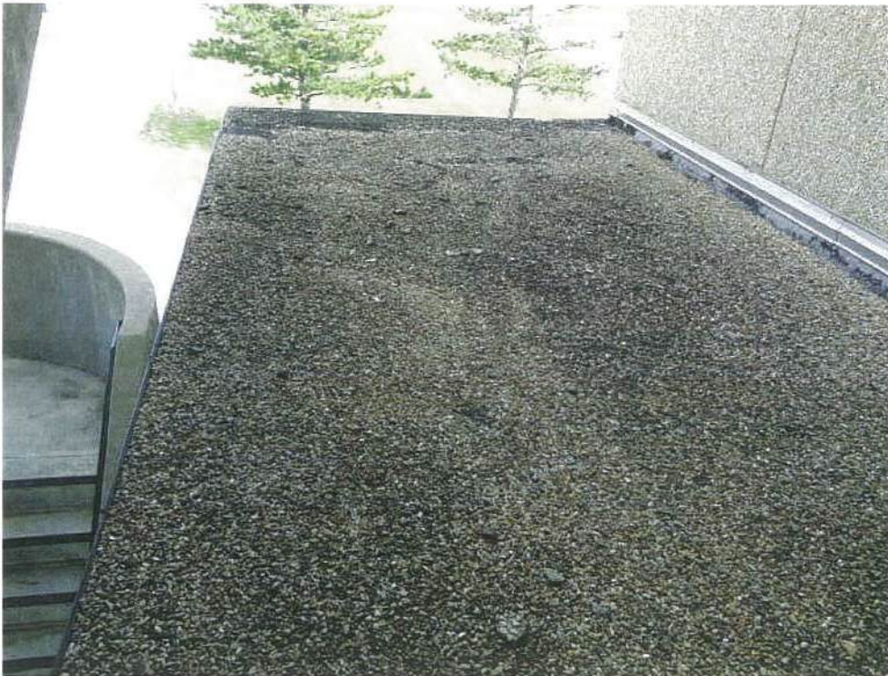
Photo #2 View of Existing Canopy Roof looking north.
