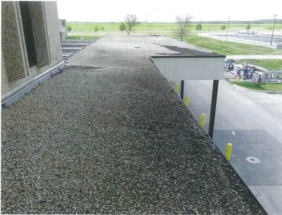
Photo #1 View of Canopy Roof looking south.
