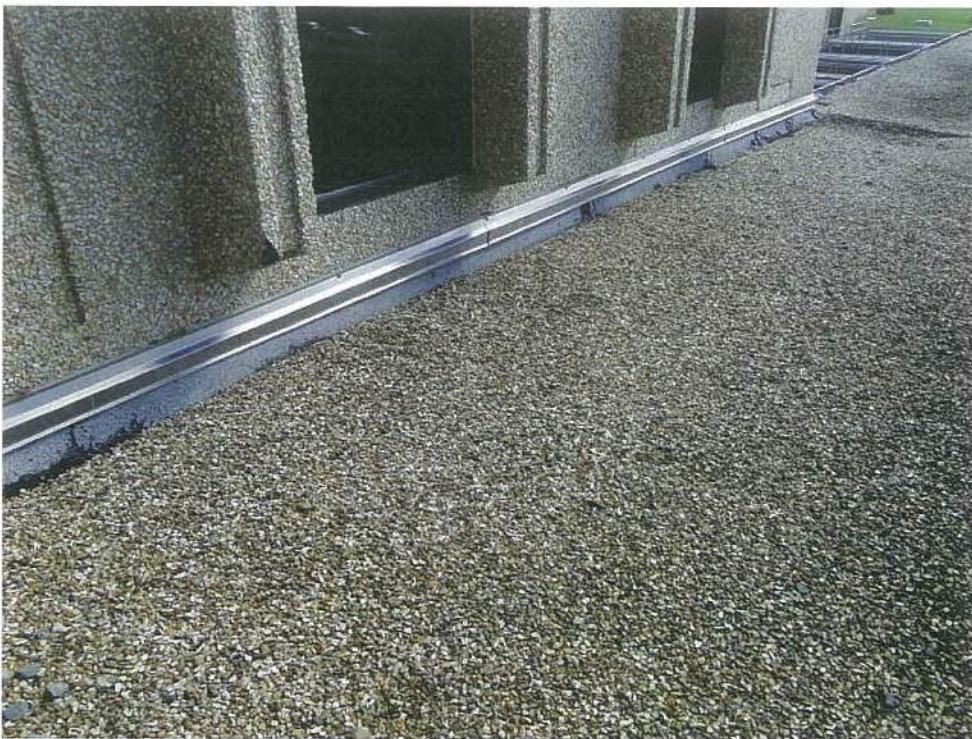
Photo #3 View of Canopy Roof looking south.
