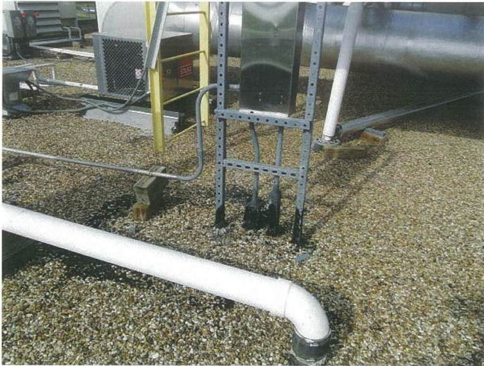
Photo #7 View of existing conduit roof penetrations & A/C equipment supports to remain at Roof Area 1.
