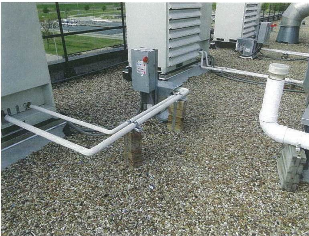
Photo #8 View of existing A/C equipment supports & pipe penetrations to remain at Roof Area 1.
