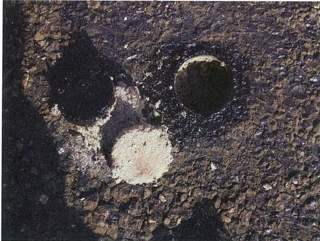
Photo #6 View of roof core cut at Bldg. B006. 1-1/2" Perlite insulation found on metal deck.
