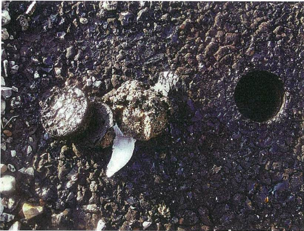
Photo #9 View of Perlite roof insulation at Bldg. B116 Roof Core Cut.
