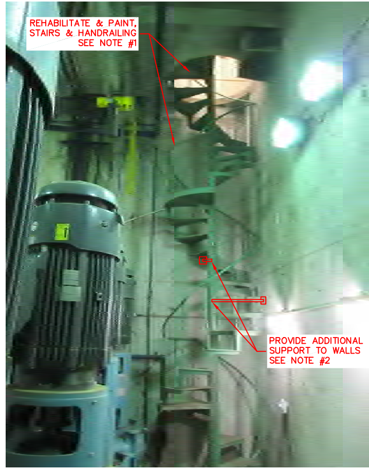
B PHOTO @ HAIKEY CREEK LIFT STATION SCALE: NTS
