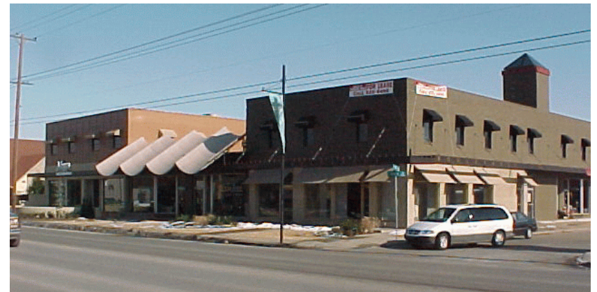
EXHIBIT F-4 - Final Construction Stage, looking northeast
