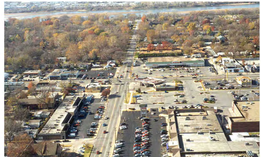
Brookside Area - 41st and Peoria, looking west
