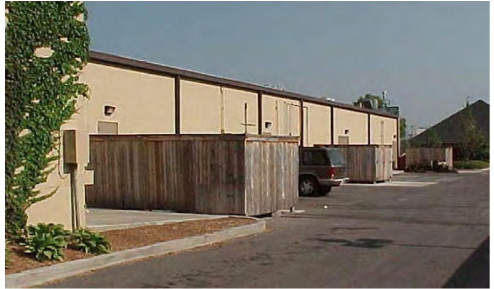
EXHIBIT I-7 - Wood screening fences with base-rail and cap-rail, located behind strip commercial center on southeast corner of 43 rd Court and S. Peoria Avenue.
