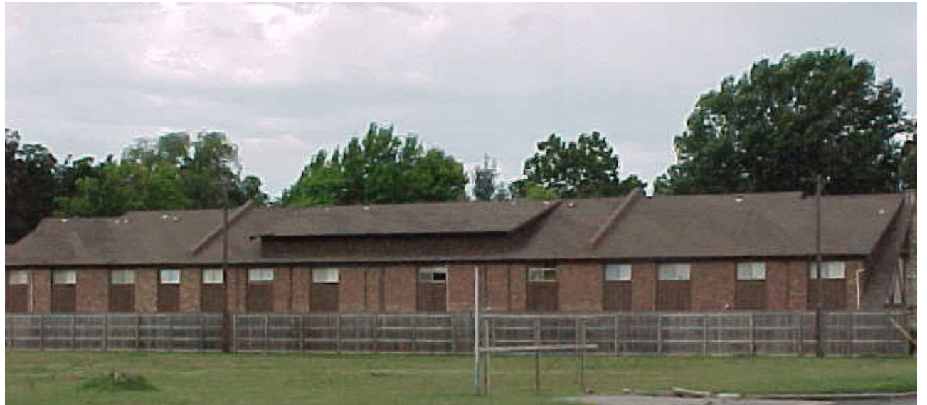
EXHIBIT L-5 - Wood fence screening only, inadequate screening, located south side of 41 st Street South near Rockford Avenue,
