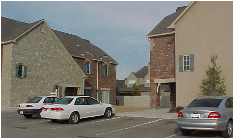
EXHIBIT G-8 - Office center behind Brooktown Shopping Center, looking east/northeast.
