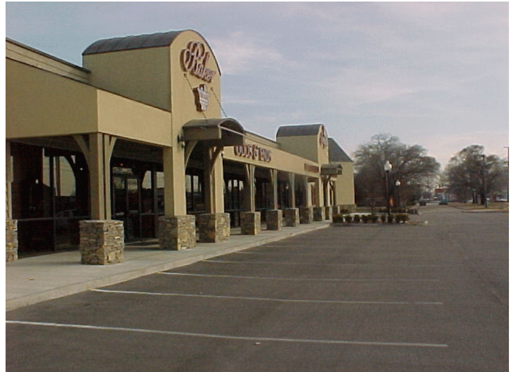
EXHIBIT G-7 - Commercial frontage and off street parking, - looking south.
