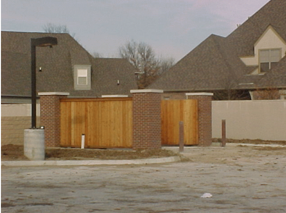
EXHIBIT I-5 - Screening fence with cap-rail, base-rail and brick pilasters -located behind Mid First Bank, Brooktown Development, at the northeast corner of 43 rd Court and S. Peoria Avenue.
