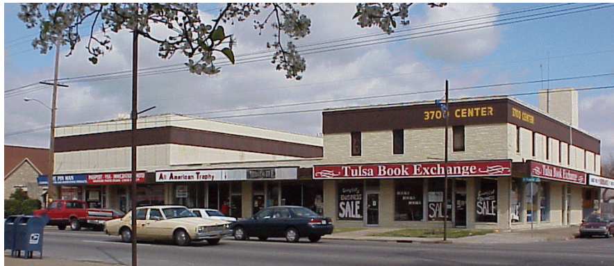
EXHIBIT F-1 - Original Conditions, looking east/northeast
