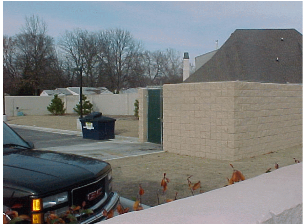
EXHIBIT I-6 - Masonry fence located behind Tulsa Auto Collection, Brooktown Development, northeast corner of 43 rd Court and S. Peoria Avenue.
