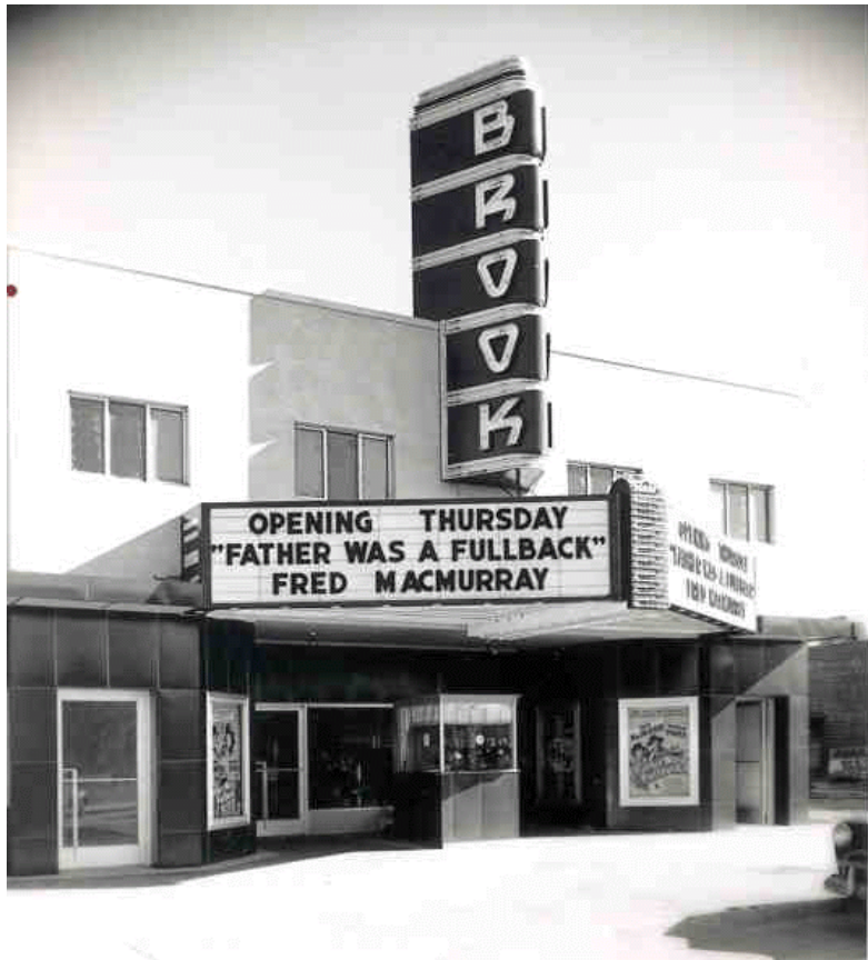
EXHIBIT E-2 - Brook Theater original conditions, looking east/southeast, 1949-50.
