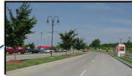
Complex entry from 193rd E. Avenue
