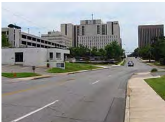
South Utica Avenue serves regional through traffic as well as the St. John Medical Center. Pedestrians on the sidewalk are unprotected from the adjoining traffic.
