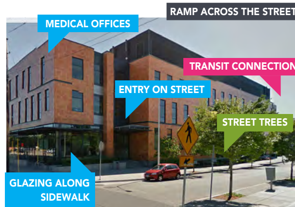
Example of an office building that creates a walkable environment with its ground-floor elements and landscaping.
