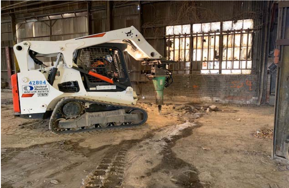
3. Concrete breaking inside Fintube building (SSD04, looking north).
