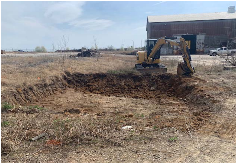
10. Excavation work in SSD12 (looking south).
