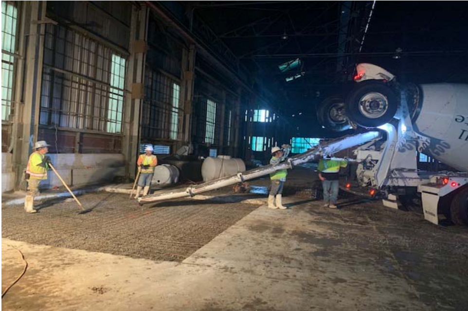
11. Concrete surface work at SSD14 (looking west).
