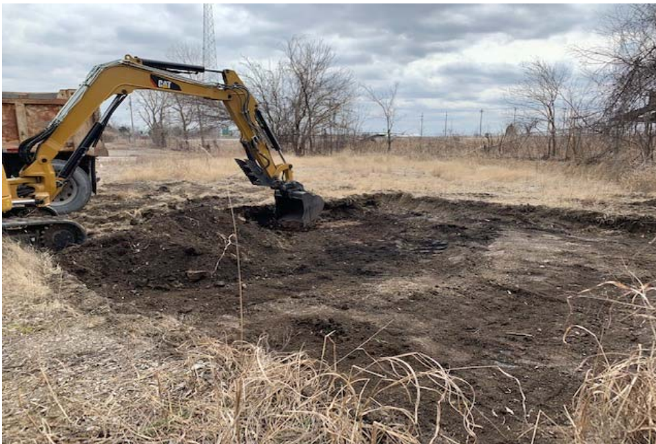
4. Excavating at SB05-SS01 (looking southwest).
