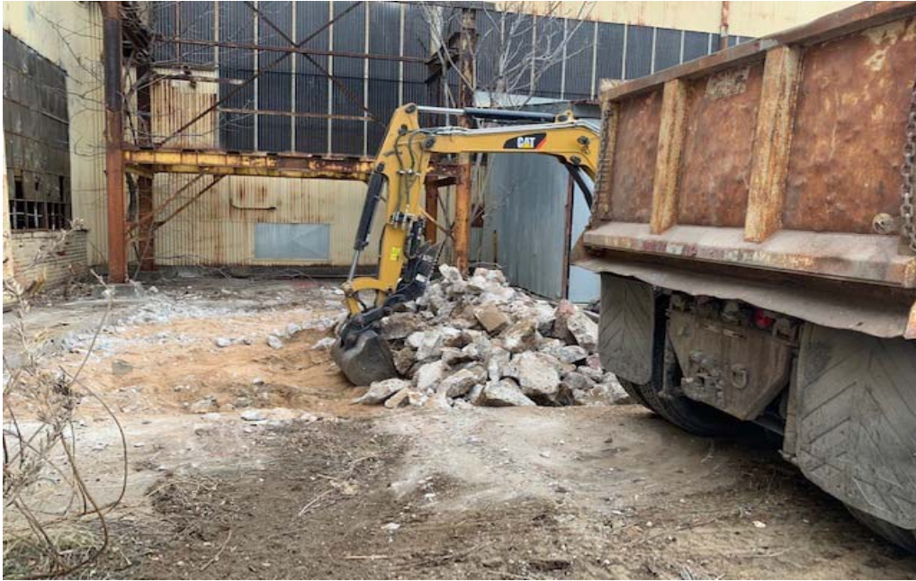
5. Removing concrete at SSD05 (looking east).
