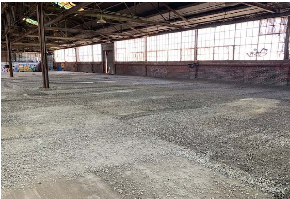
8. Floor brick pavers area in Evans building following gravel backfill (looking northeast).
