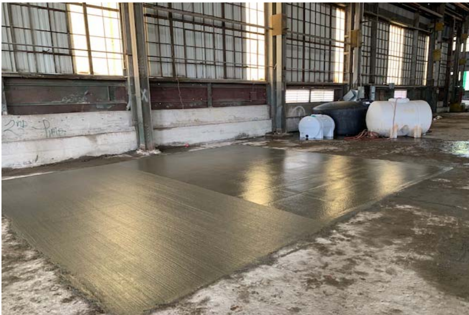
12. Final concrete surface at SSD14 (looking southwest).
