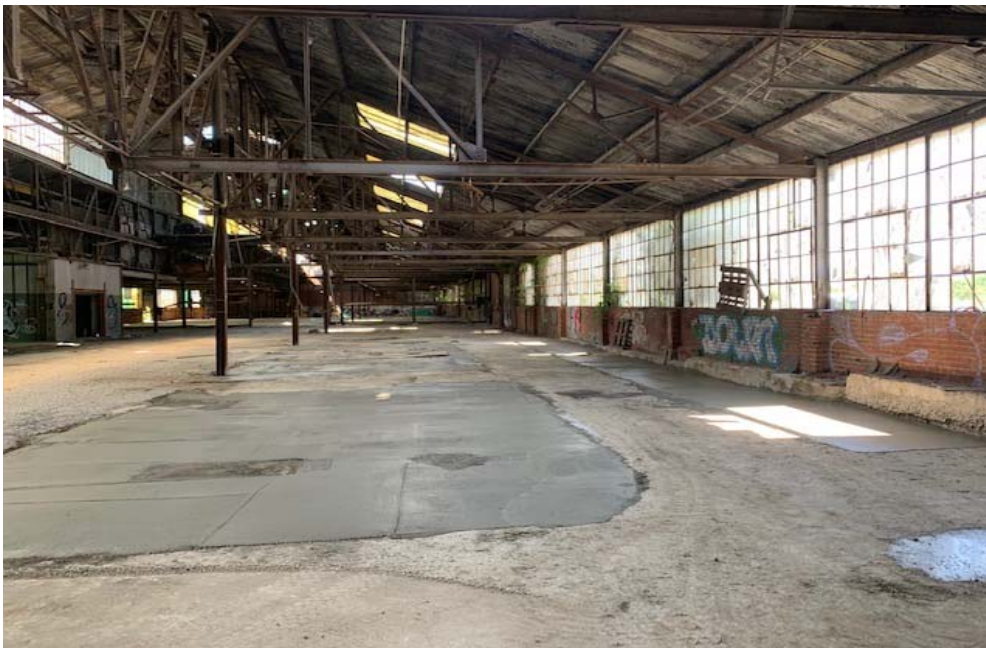
14. Final concrete surface in floor brick pavers area (looking north).
