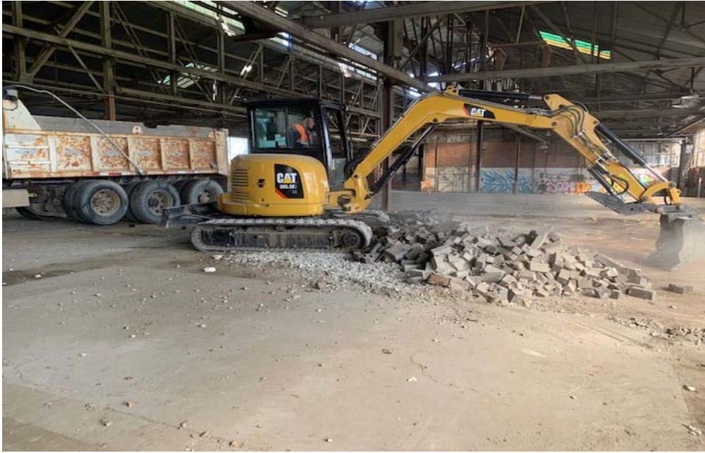
1. Removal of floor brick pavers inside Evans building (looking north).
