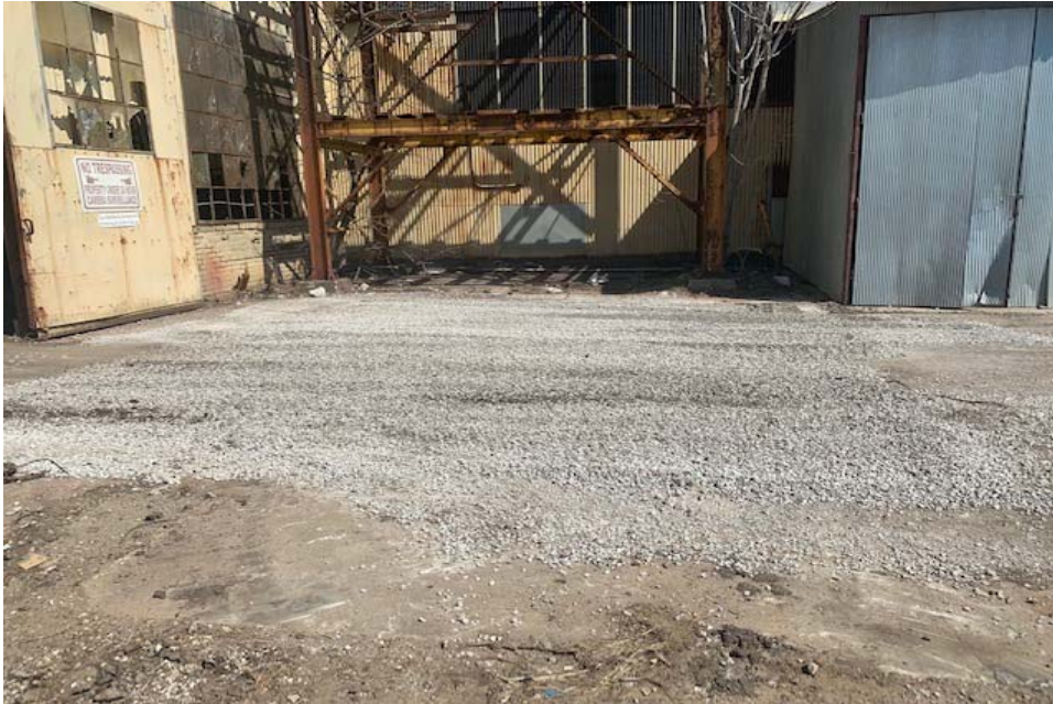
9. SSD05 following excavation and backfill activities (looking east).
