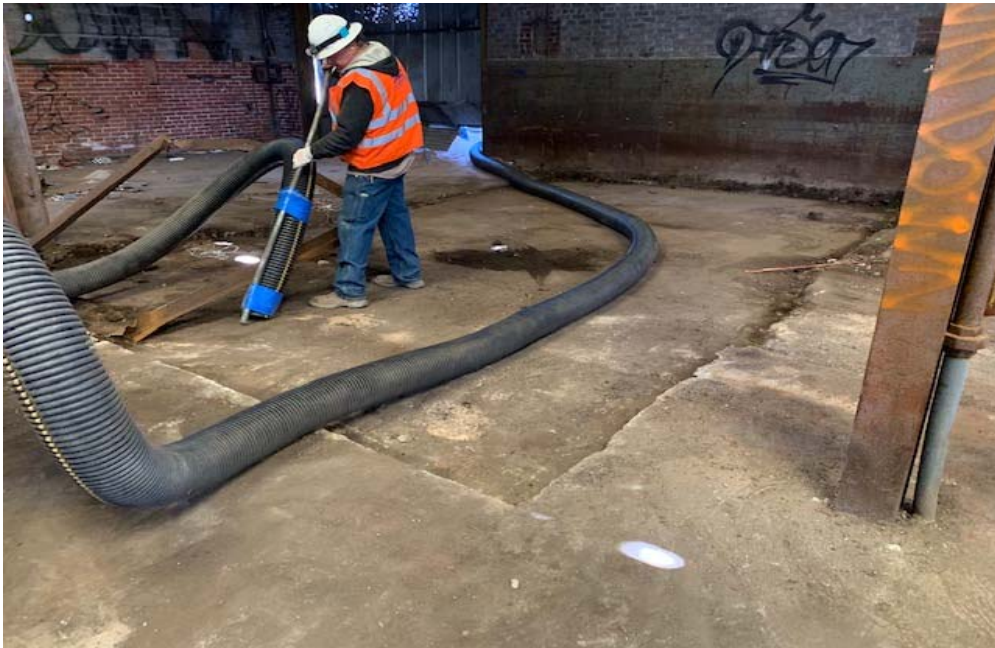
2. Removal of floor brick pavers inside Evans building with Guzzler air mover.
