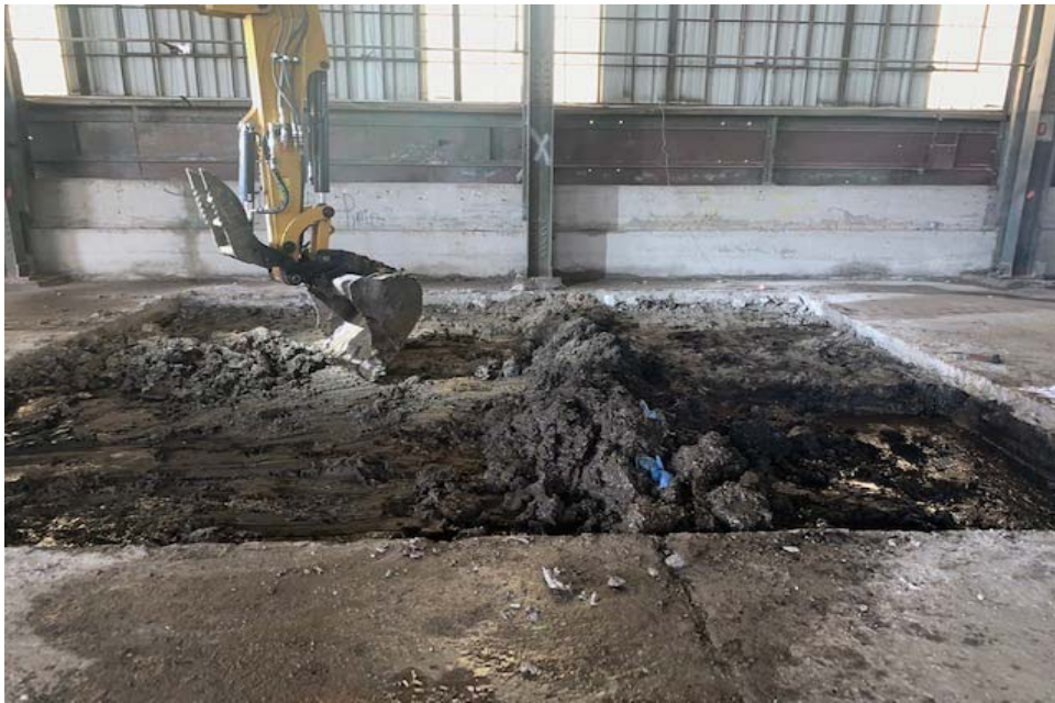
6. Excavation at SSD14 (looking south).
