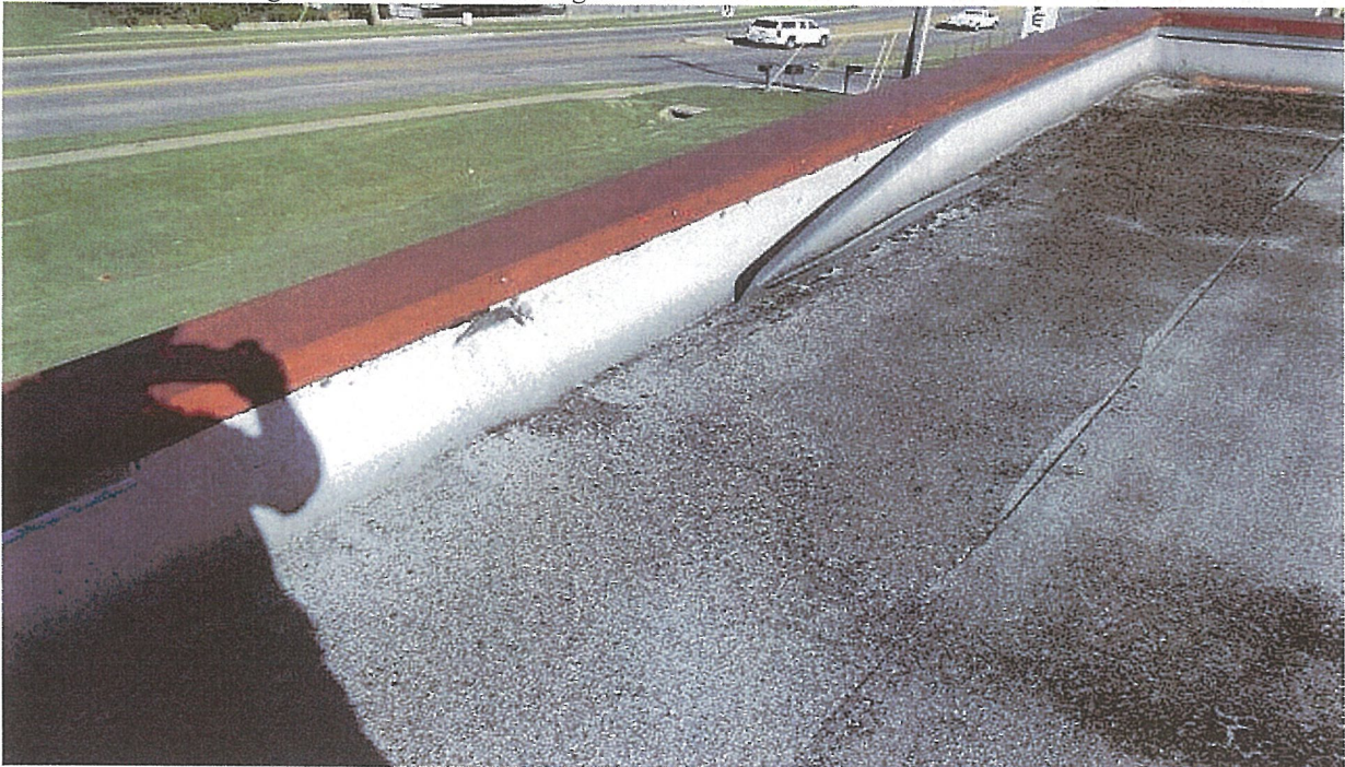
Photo 10 View of existing metal coping at the west parapet wall of the west building.
