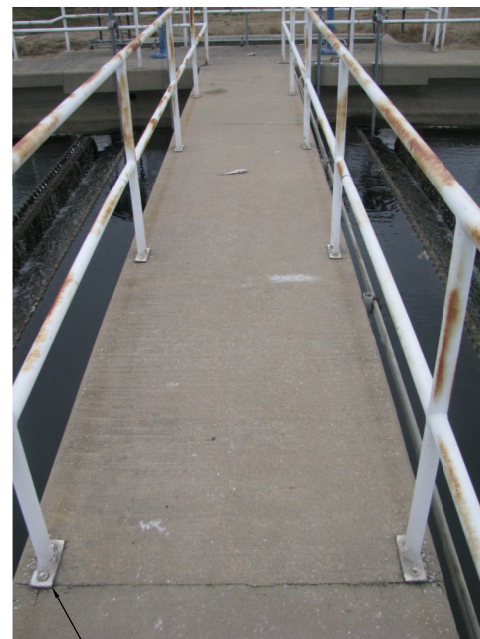
NEW RAILING POST SHALL BE INSTALLED AFTER THE REPAIR, AND THE POST ANCHOR BOLT SHALL BE AT LEAST 9" AWAY FROM THE REPAIRED CRACK
