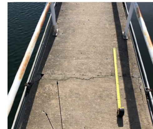
REPAIR THE CRACK ON HORIZONTAL SURFACE REPAIR THE DEFICIENT SURFACE AREA
