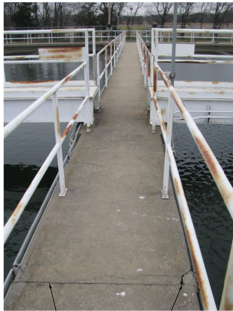
HORIZONTAL SURFACE REPAIR CRACK AT EDGE OF WALKWAY, COMBINED HORIZONTAL AND VERTICAL REPAIR
