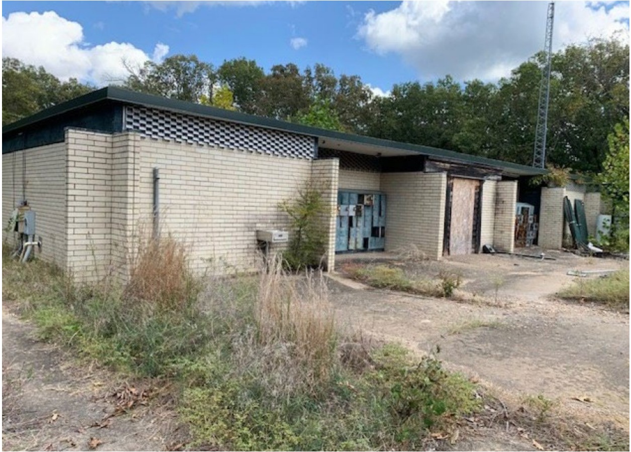
Rear of office and lockers for former swimming pool that has been filled in (looking northeast)
