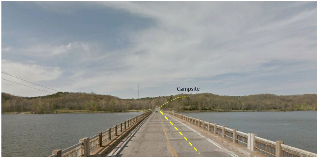
Bridge road to campsite location (looking north)
