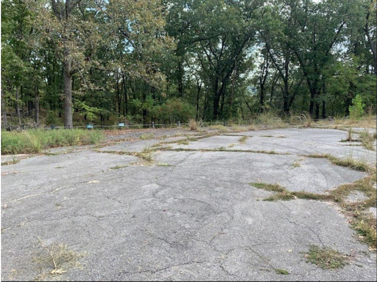
Paved area at top of hill (looking east)
