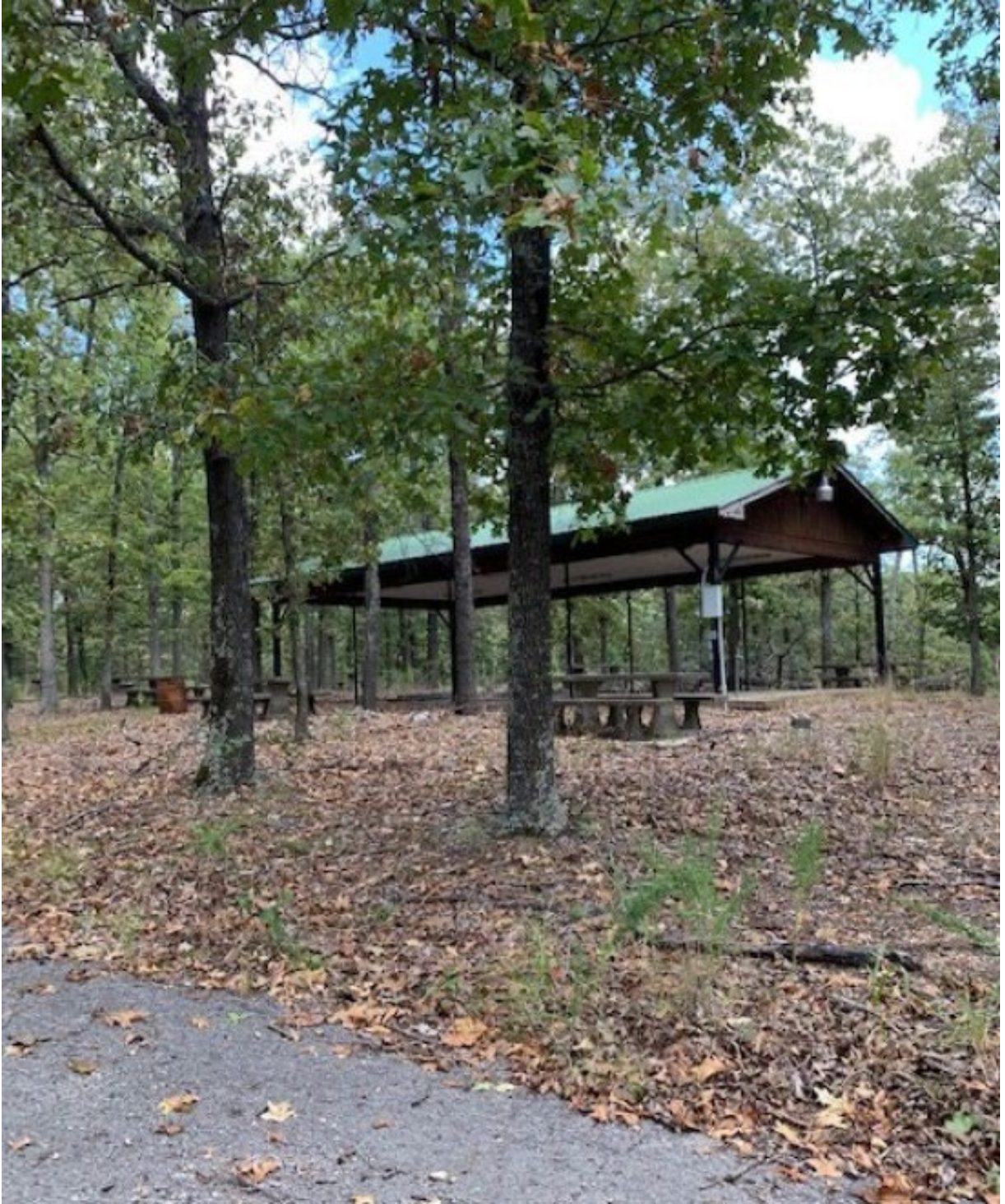
Camp Pavilion (looking northeast)
