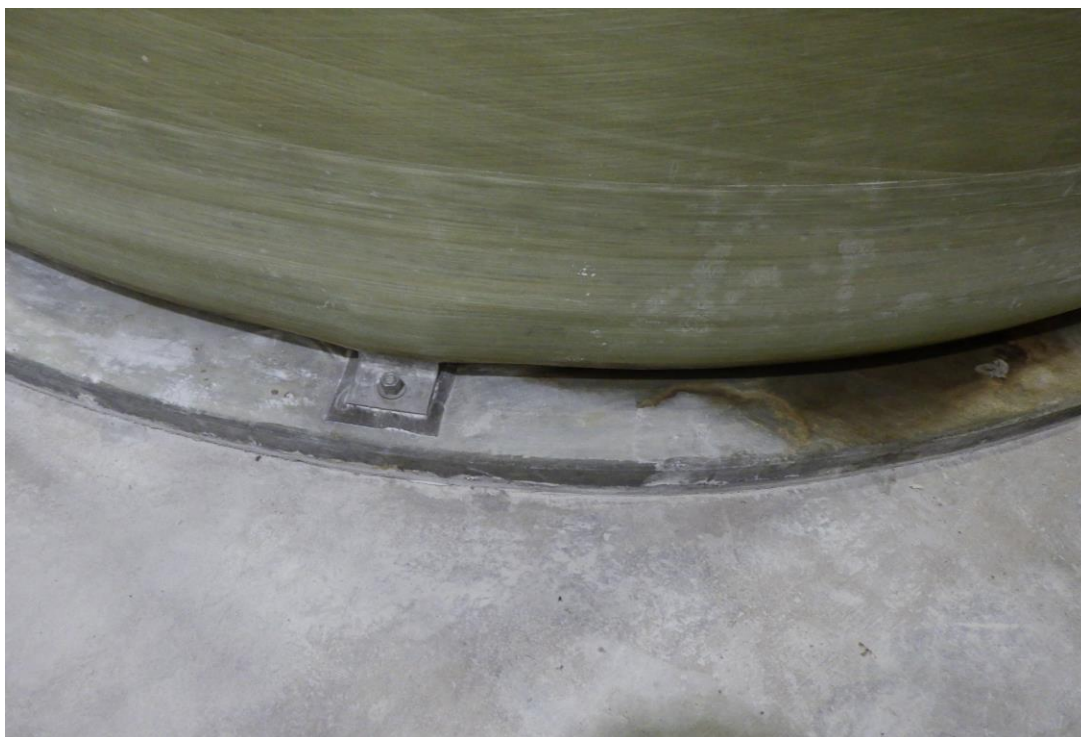
PHOTO #6 – TYPICAL APPEARANCE OF FOUNDATION BOLTS
