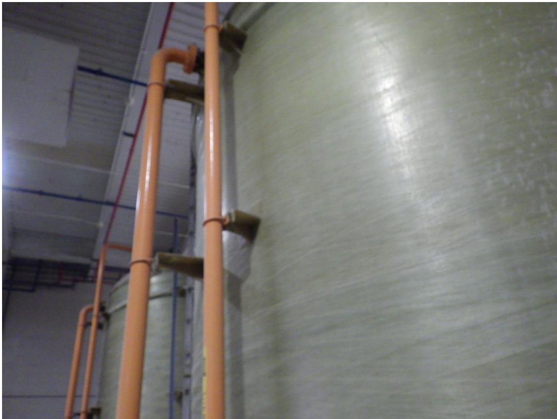
PHOTO #* – TYPICAL APPEARANCE OF STAND-OFFS AND ATTACHMENTS
