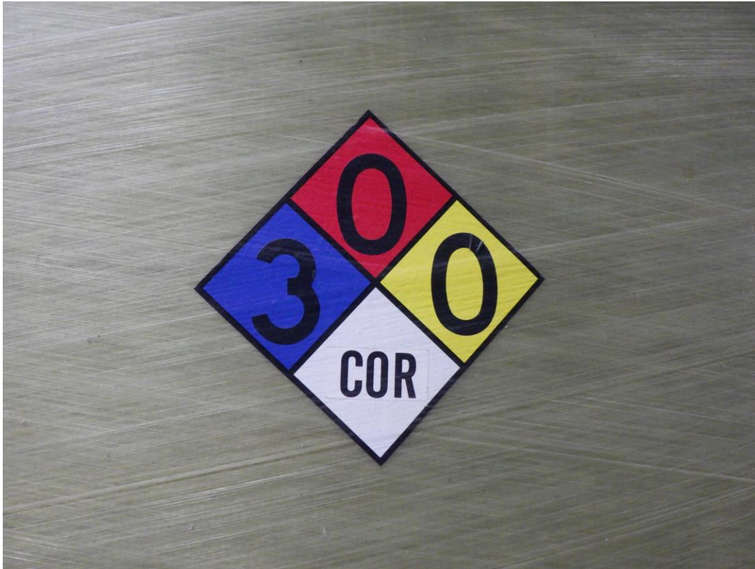
PHOTO #2 – NFPA LABELS AND HAZARD WARNINGS VISIBLE ON TANK
