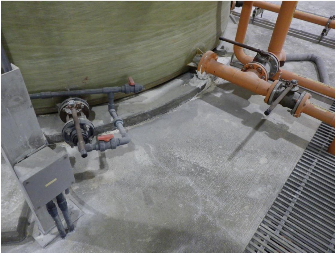
PHOTO #9 – LEAK ON THE DRAIN NOZZLE
