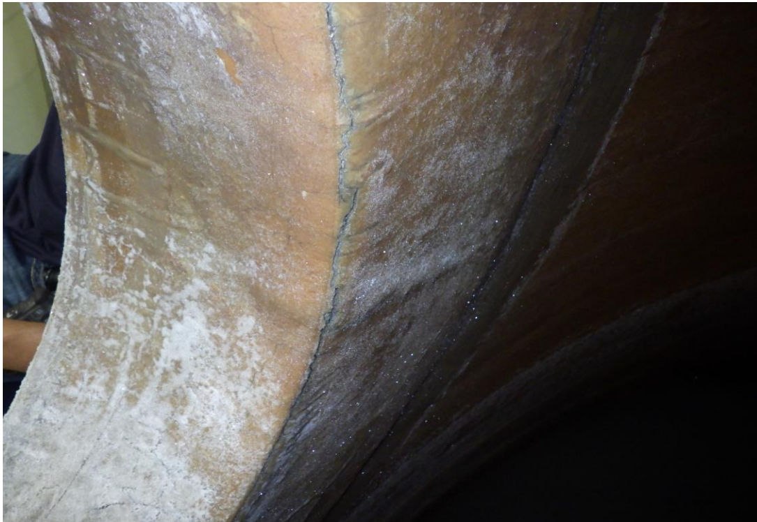
PHOTO #12 – OVERALL VIEW OF THE CRACK INDICATIONS IN THE MANWAY
