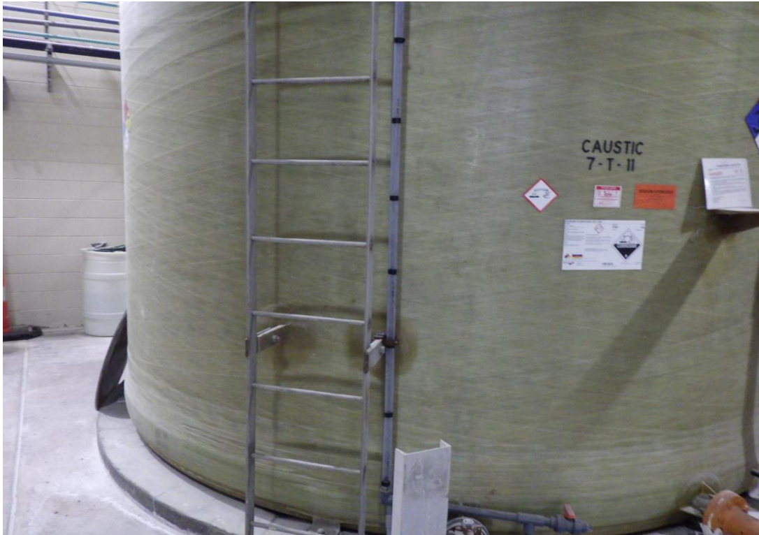
PHOTO #7 – TANK LEVEL GAGE ADJACENT TO LADDER
