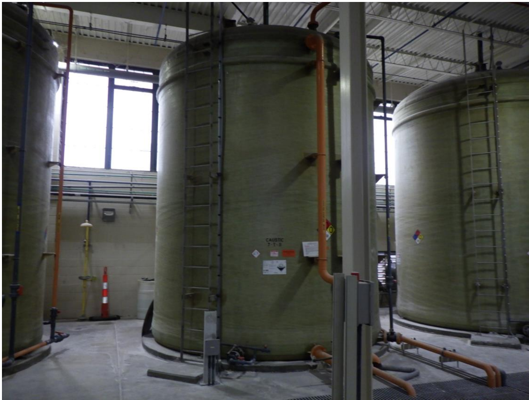
PHOTO #1 – OVERALL VIEW OF TANK 7 – T – 11
