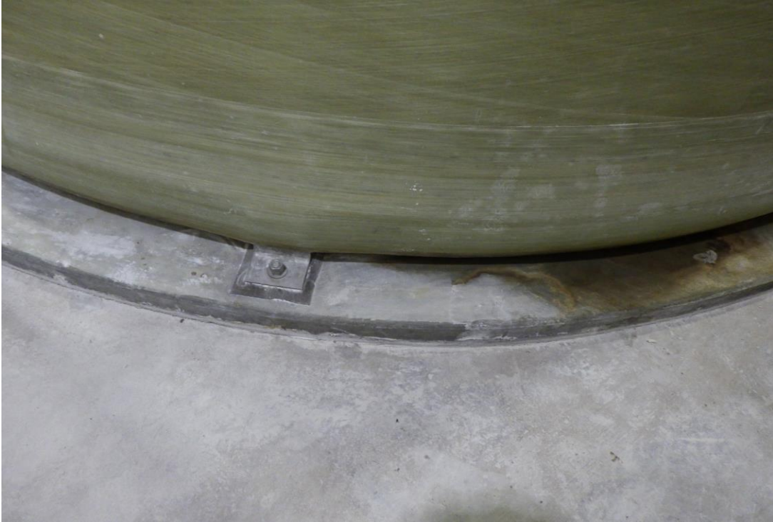
PHOTO #6 – TYPICAL APPEARANCE OF FOUNDATION BOLTS
