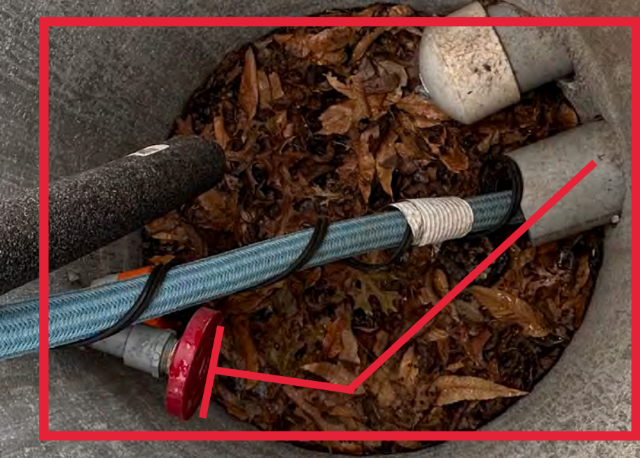
SOUTH BASIN TYPICAL CONNECTION POINT OF TUBING
