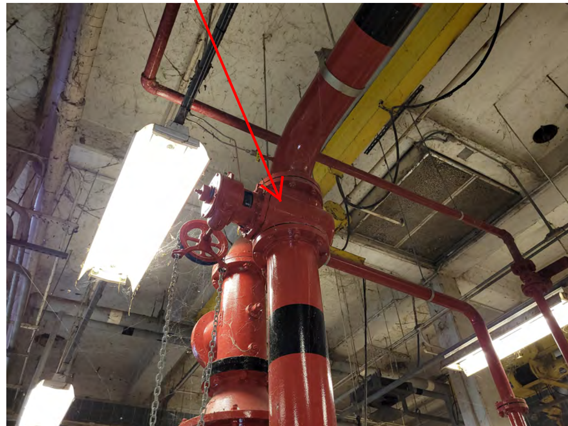
Valve to Boiler 3
