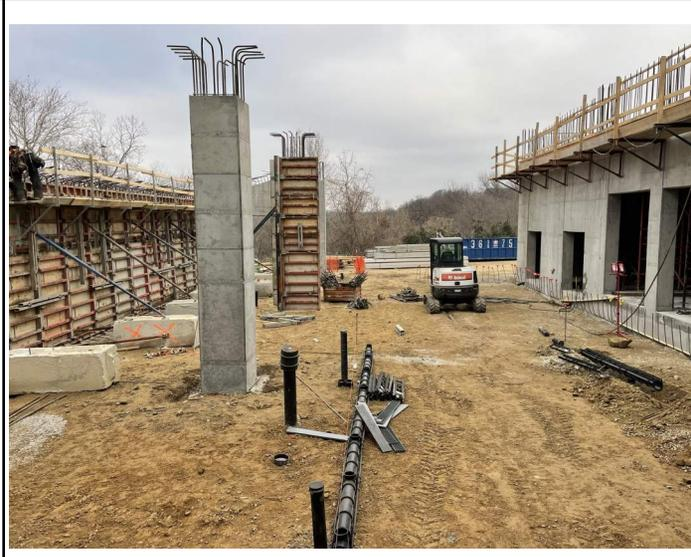
Trench drains are being installed before SOG pour at the loading dock.
