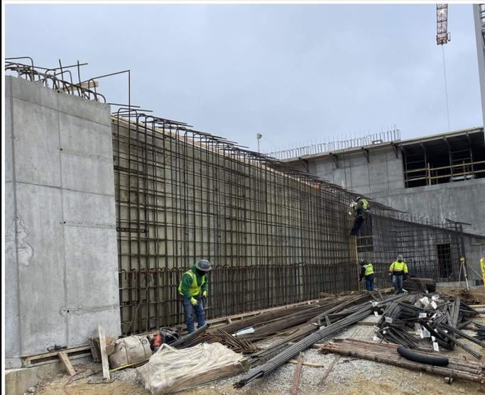
Wall along GL D in the loading dock is formed and the north half is being poured today.
