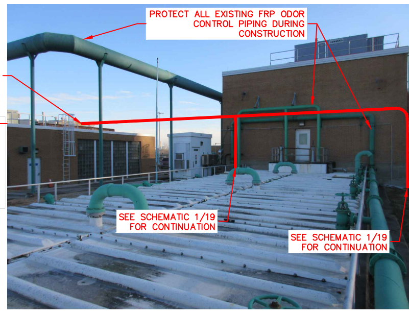
A 20 PHOTO - EXISTING BLOWER & ODOR CONTROL PIPING SCALE: NTS
