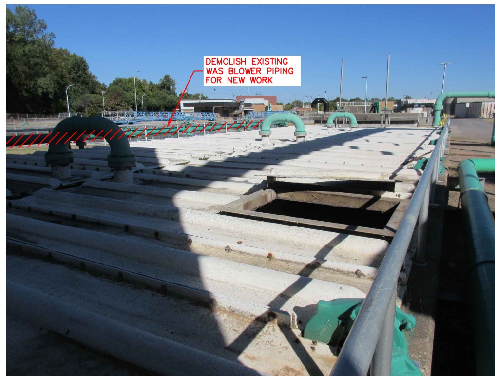
D PHOTO — EXISTING BLOWER & ODOR CONTROL PIPING SCALE: NTS
