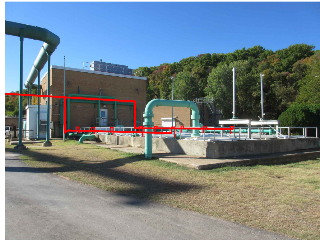
B PHOTO — EXISTING BLOWER & ODOR CONTROL PIPING 22 SCALE: NTS
