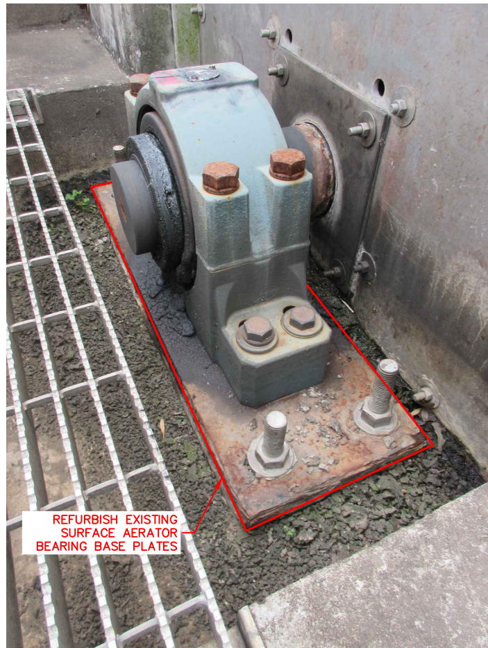
1 PHOTO — EXISTING SURFACE AERATOR BEARING 38 SCALE: NTS
