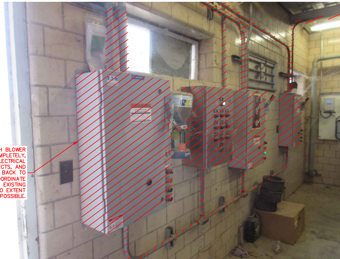
C PHOTO – EXISTING BLOWER ROOM (LOOKING SOUTH) 16 SCALE: NTS
