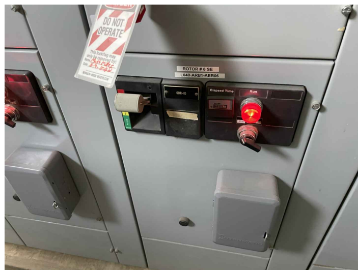
EXISTING STARTER TO BE REMOVED SCALE: NONE
