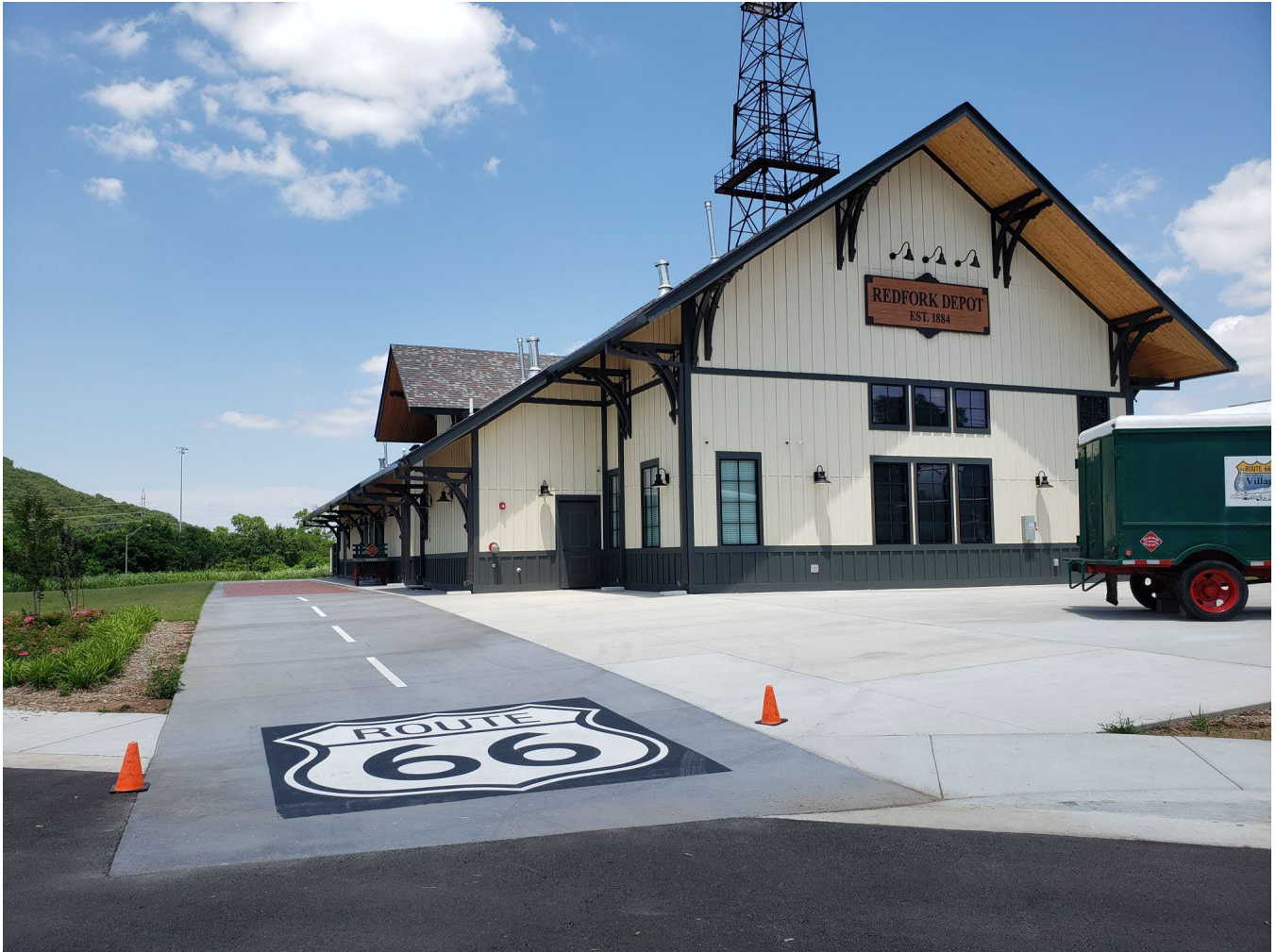
Figure 2: Looking east at the entrance to the Train Depot showing the replica of the Route 66 Highway
