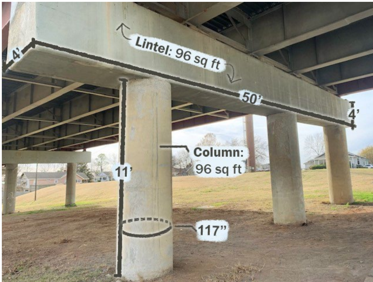
Figure 2: Column and Lintel Measurements
