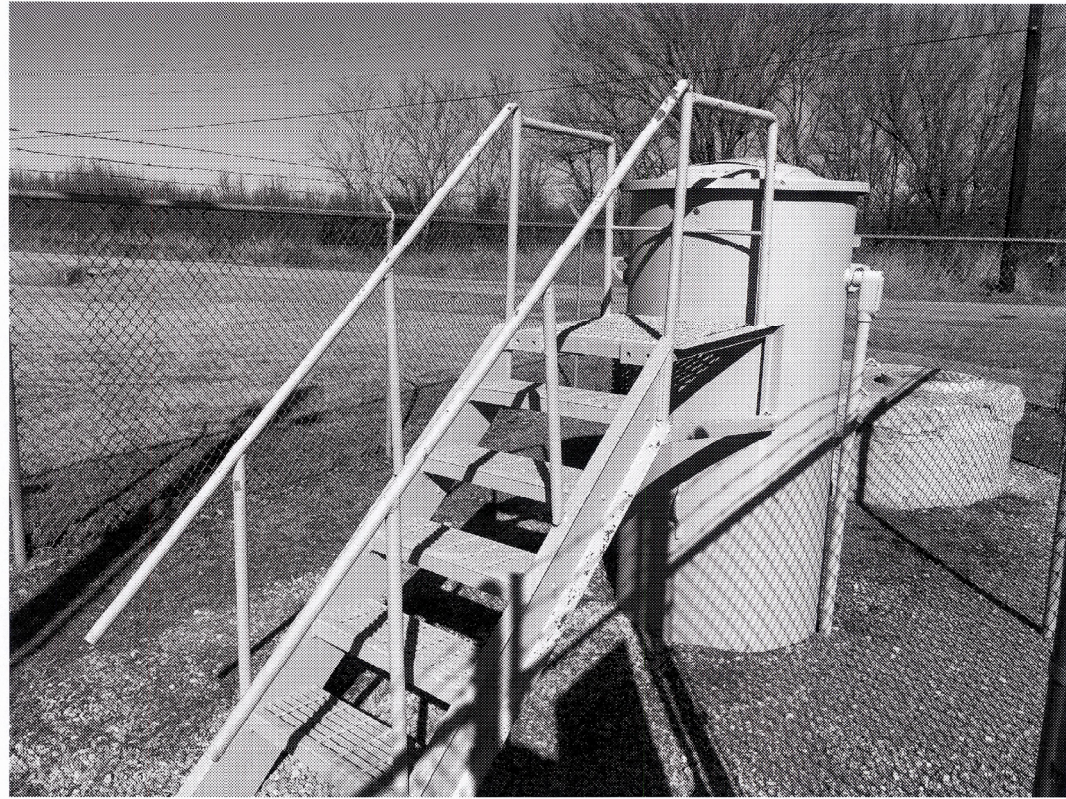
1 PHOTO — EXISTING LIFT STATION 18 NTS
