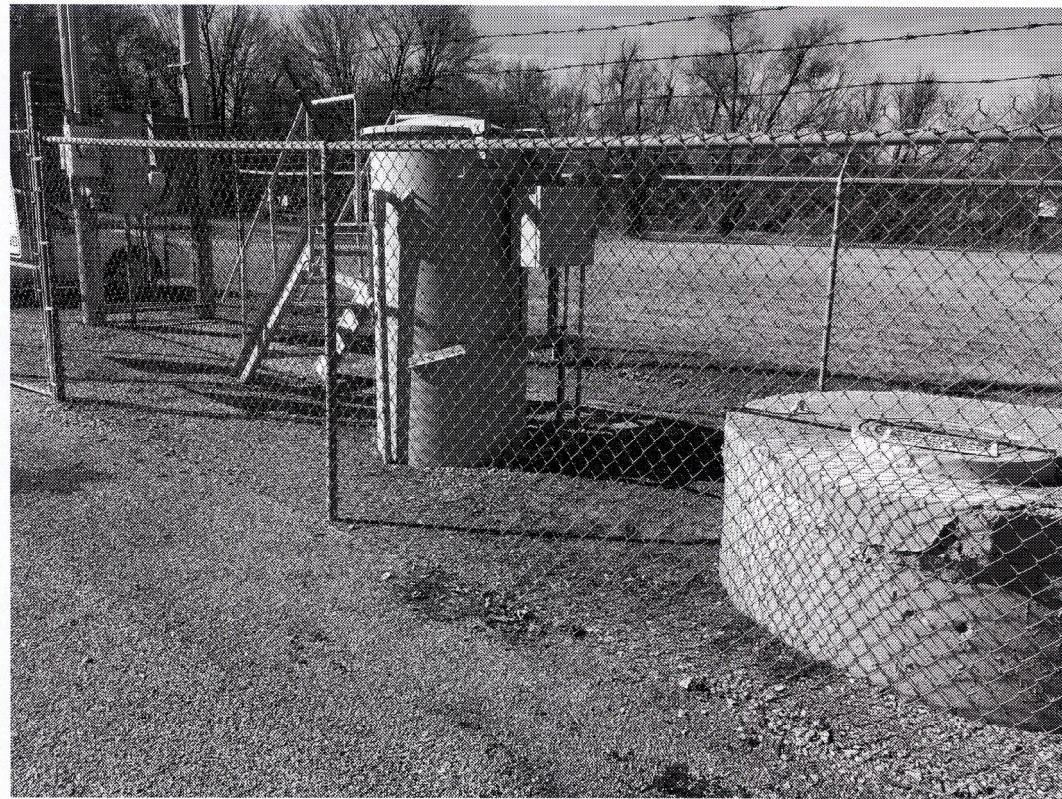
2 PHOTO — EXISTING LIFT STATION 18 NTS
