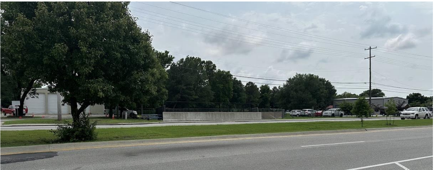
Figure 3: Photo of Eastbound Wall of Bridge #247
