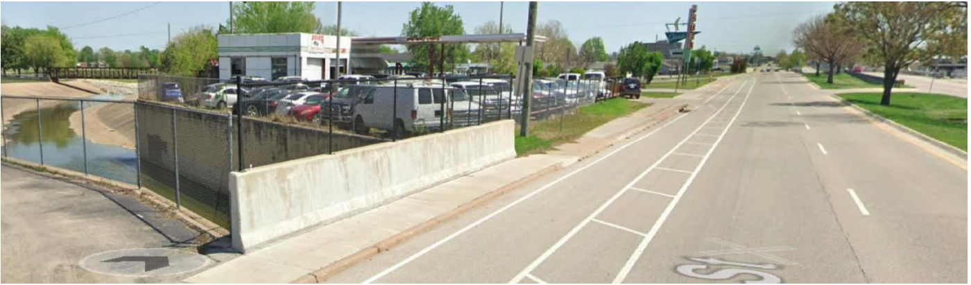
Figure 2: Photo of Westbound Wall of Bridge #247
