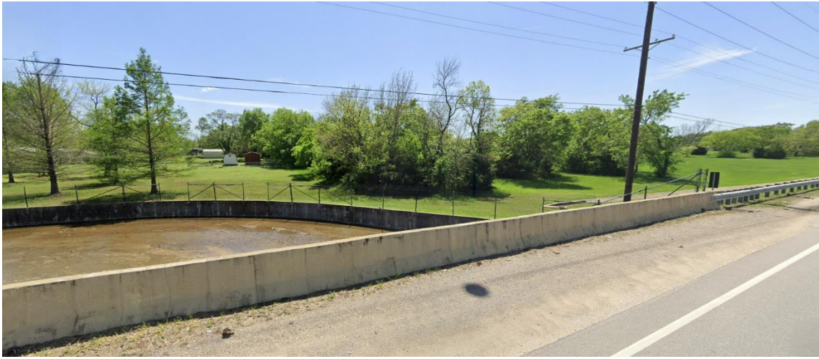
Figure 2: Photo of Westbound Wall of Bridge #251
