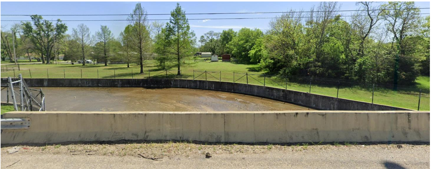
Figure 3: Photo of Eastbound Wall of Bridge #251
