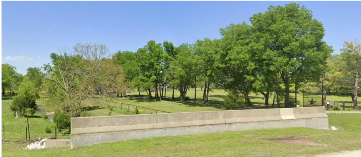
Figure 2: Photo of Westbound Wall of Bridge #252
