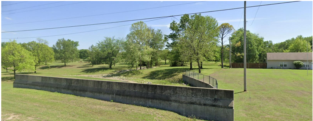
Figure 3: Photo of Eastbound Wall of Bridge #252
