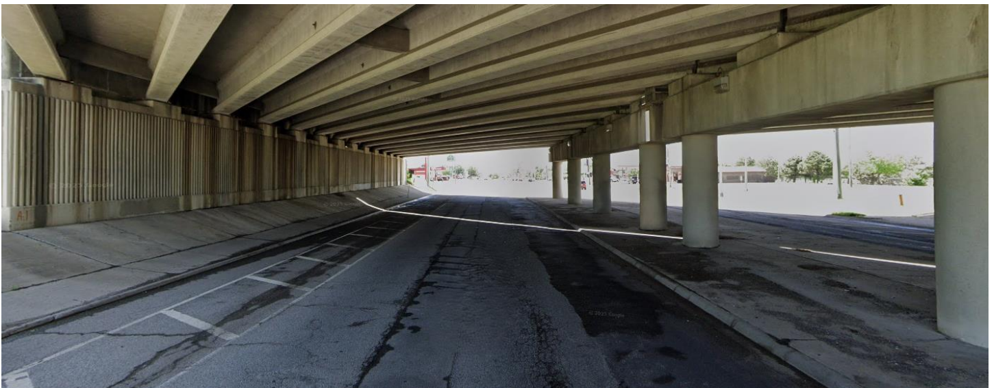
Figure 3: Photo of Eastbound Wall and Pillars of I-44 Highway Underpass
