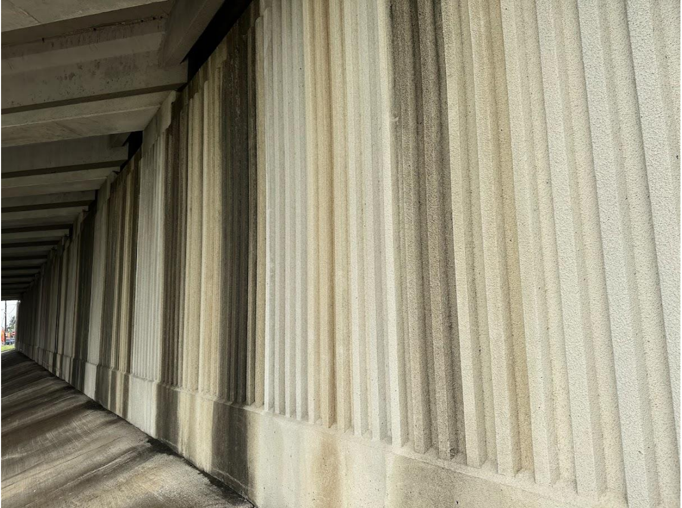
Figure 4: Photo of Ridged Surface of I-44 Highway Underpass
