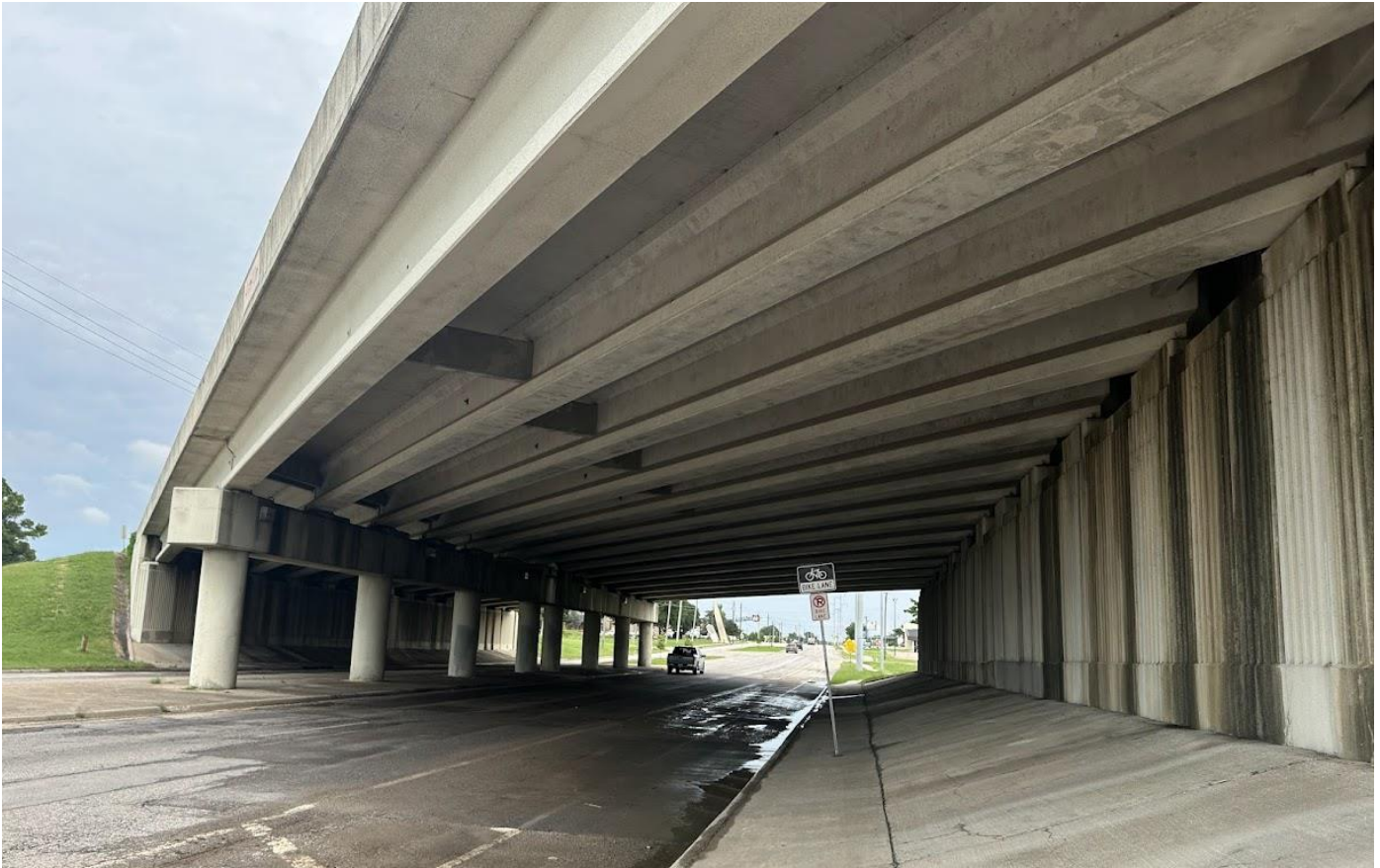
Figure 2: Photo of Westbound Wall of I-44 Highway Underpass
