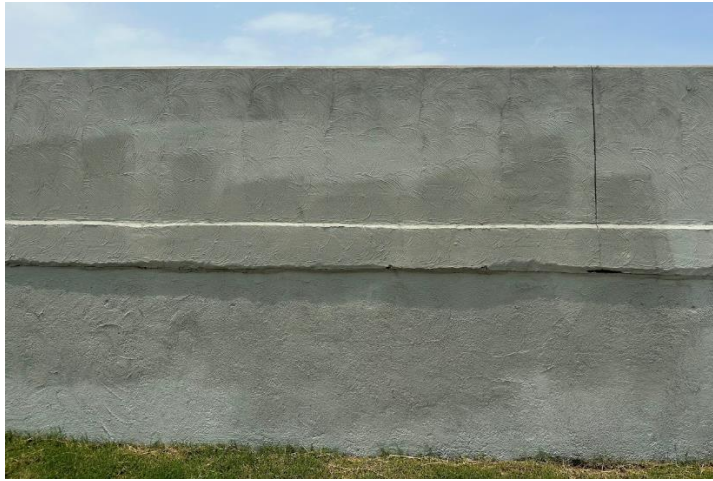
Figure 2: Closeup Photo of US-75 Highway Retaining Wall
