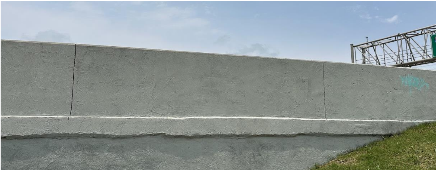
Figure 3: Photo of US-75 Highway Retaining Wall
