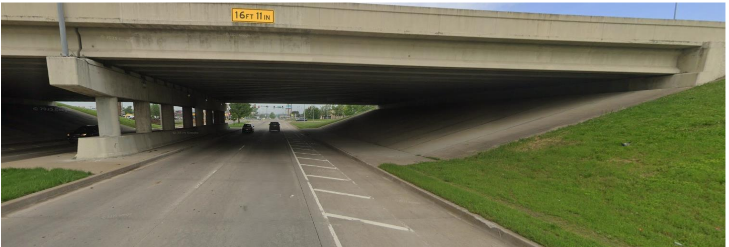
Figure 3: Photo of Westbound Wall and Pillars of I-169 Highway Underpass
