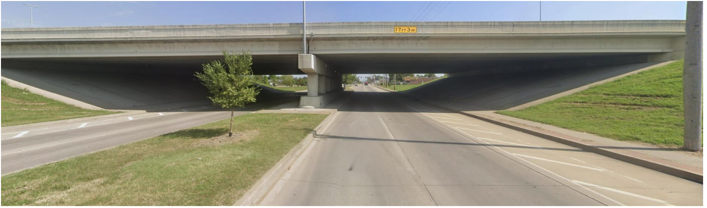
Figure 2: Photo of East- and Westbound Wall of I-169 Highway Underpass
