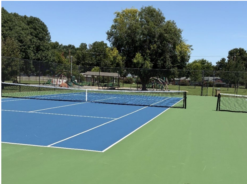
Darlington Park Tennis Court (Project 5)
