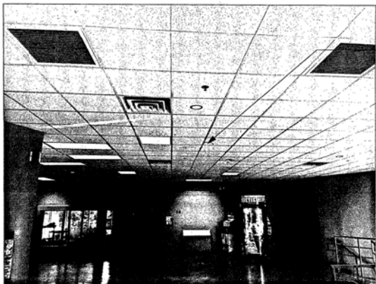
F EXISTING CONDITIONS PHOTO- ARCTIC CEILING 1 1/2" = 1'-0"
