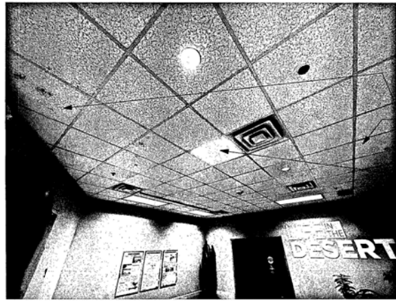
G EXISTING CONDITIONS PHOTO- DESERT CEILING 1 1/2" = 1'-0"
