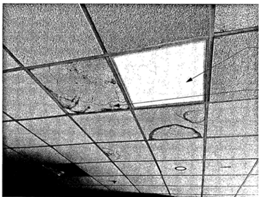
D EXISTING CONDITIONS PHOTO- ARCTIC CEILING 1 1/2" = 1'-0"
