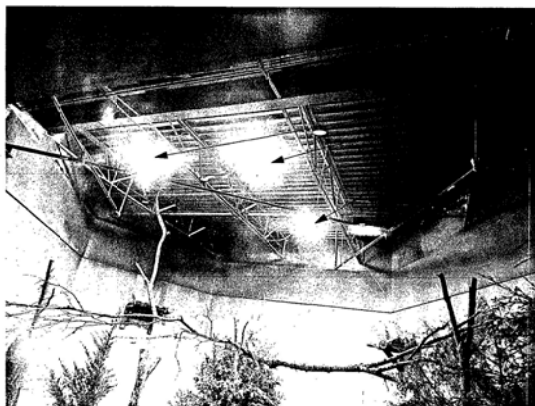
E EXISTING CONDITIONS PHOTO- ARCTIC CEILING 1 1/2" = 1'-0"
