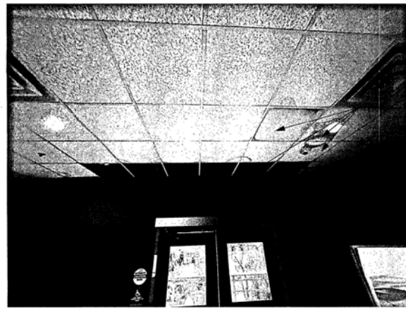
F EXISTING CONDITIONS PHOTO- DESERT CEILING 1 1/2" = 1'-0"
