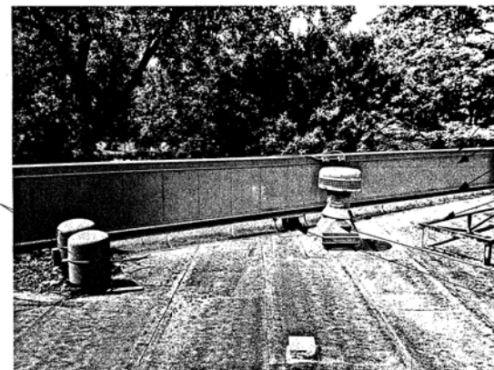
C EXISTING CONDITIONS PHOTO- FOREST ROOF 12" = 1'-0"
