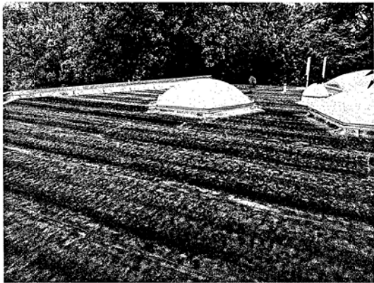
F EXISTING CONDITIONS PHOTO- FOREST ROOF 12" = 1'-0"
