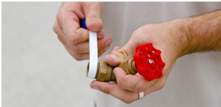
Prepare the threaded side of the 3/4" faucet by wrapping it tightly with Teflon tape (make four or five rotations until all the threads are covered) or apply a thin bead of silicone caulk around the threads.
