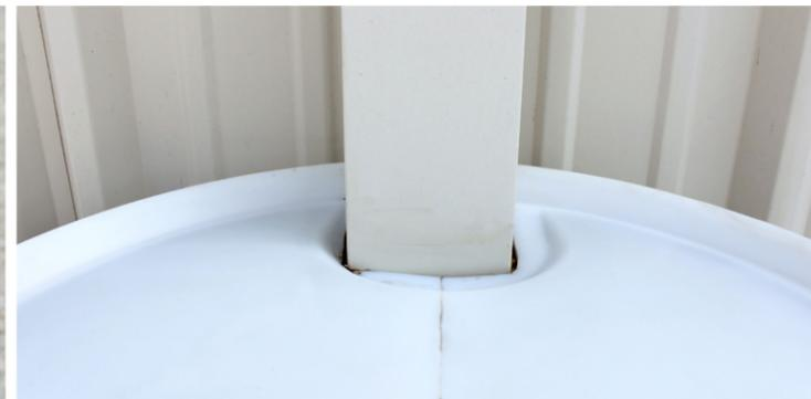
Cut your downspout about 4" above the top of the barrel, add the elbow from the bottom of the downspout and insert it into the freshly cut gutter downspout.
