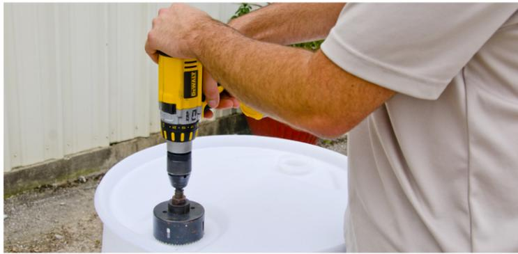
Use a 6" hole saw to cut a round 6" hole in the lid of your barrel.
