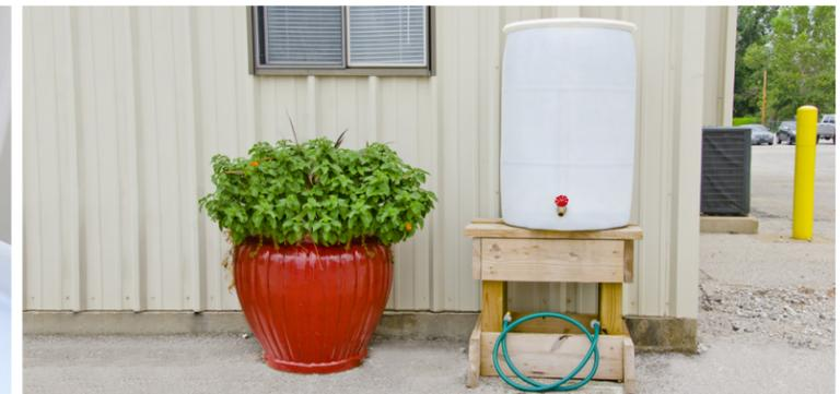
Place a wooden stand or two cinder blocks under the selected downspout and place the barrel on this raised base. Make any final adjustments to the base and barrel to make it level.
