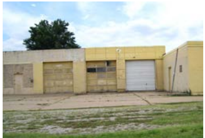
Vacant commercial building
