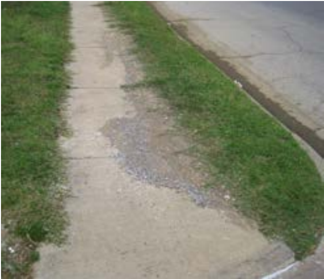
Sidewalk covered with debris
