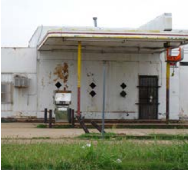
Old gas station building on Peoria Avenue ADOPTED 2013/AMENDED 2016
