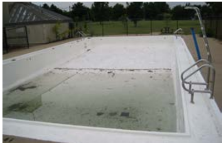
Closed pool facility at Hawthorne Park
