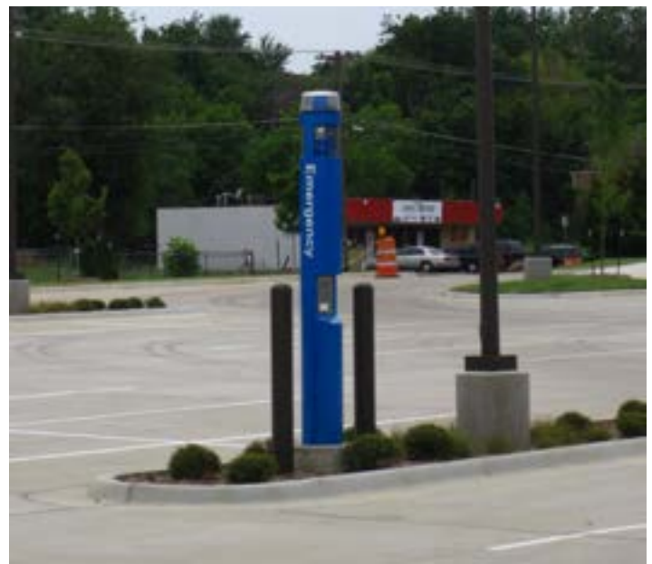
Emergency contact station
