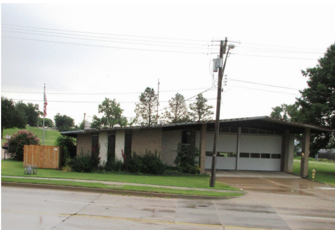
Former Fire Station #9, now Fire Administrative offices, 1420 Charles Page Boulevard.
