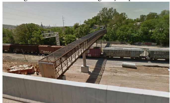
Pedestrian Bike Bridge, closed for reconstruction.
