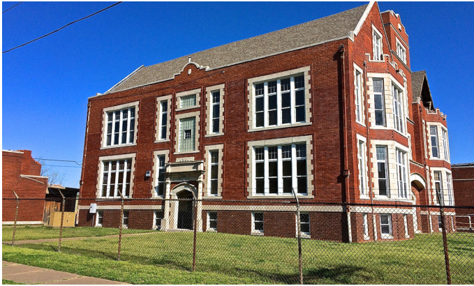
The remaining facade of the Irving School building - Maybelle Avenue at W. Archer - visibly represents the historic beginnings of Crosbie Heights.
