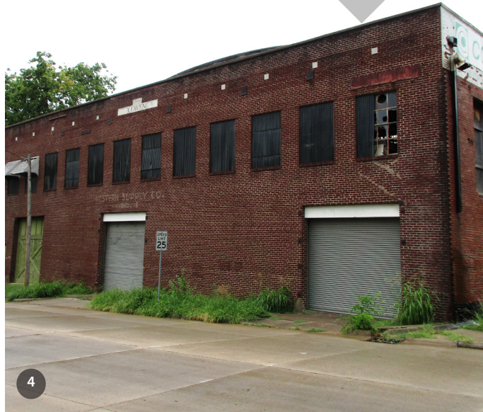
Western Supply Co. Warehouse 1928
