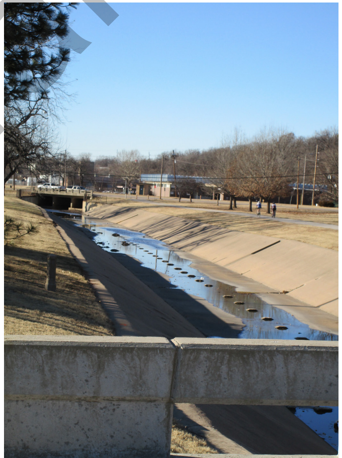
Parkview Drainage Ditch collects runoff from Crosbie Heights and neighboring areas.
