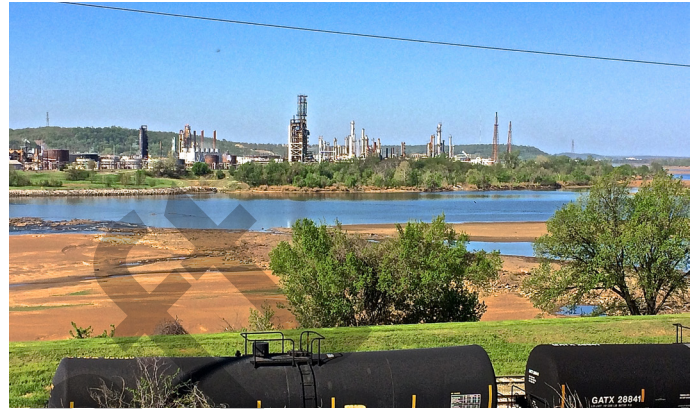
Holly/Frontier refinery, across the Arkansas River from Crosbie Heights.
