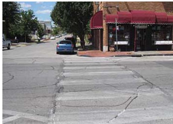
Faded cross-walk on Cherry Street (East 15th). The plan area has a shortage of well-signed, safe crossings for pedestrians.
